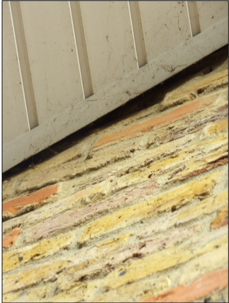
Figure 7. Gap between soffit and wall on western elevation. 216b Nine Mile Ride, Wokingham. 21.01.25
