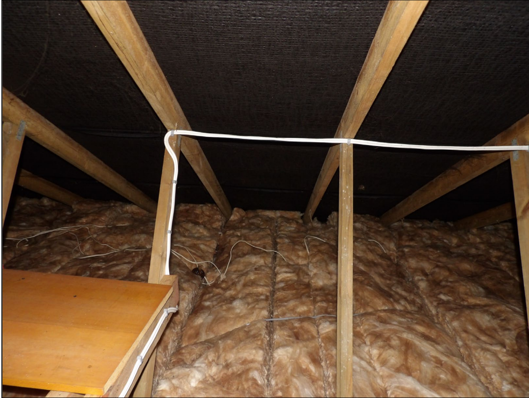
Figure 12. Example of bitumen lining in loft space. 216b Nine Mile Ride, Wokingham. 21.01.25
