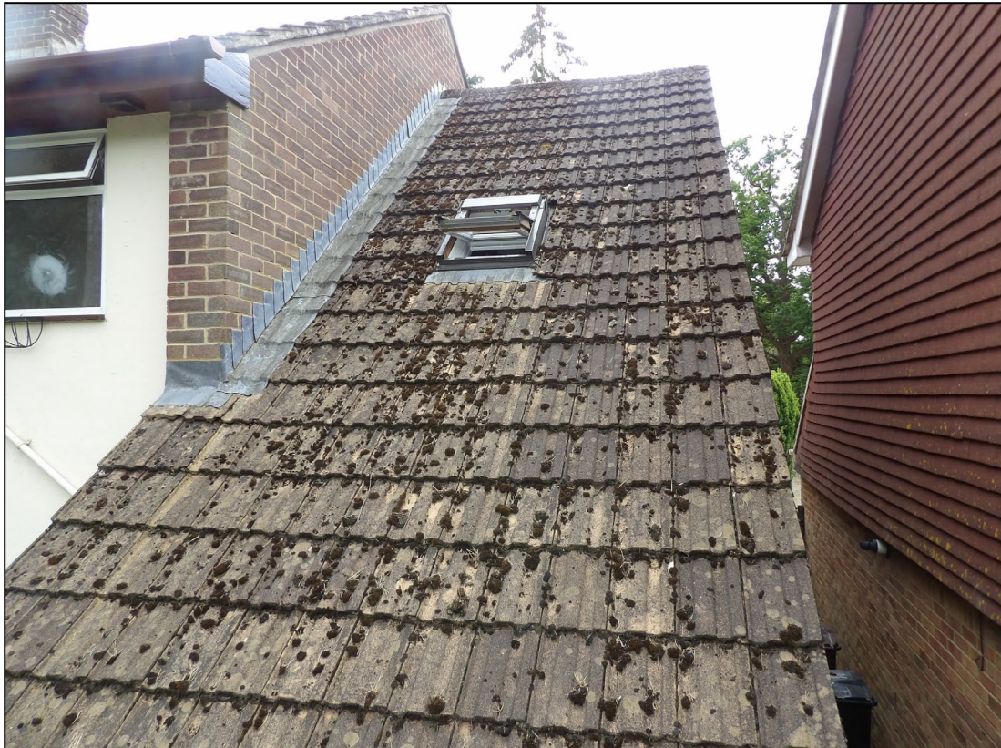
Figure 8. Example well fitted lead flashing. 104 Reading Road, Finchampstead. 10.06.25
