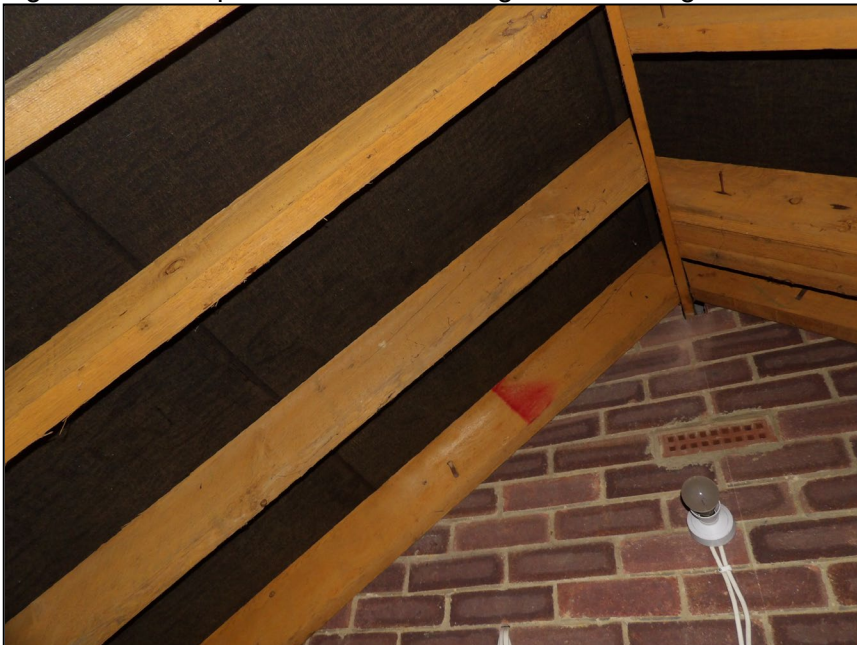
Figure 14. Example of membrane lining. 104 Reading Road, Finchampstead. 10.06.25
