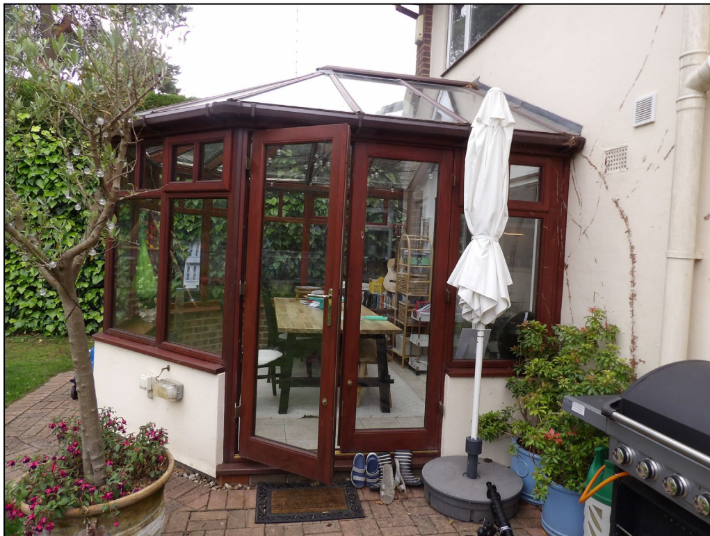
Figure 10. Rear conservatory. 104 Reading Road, Finchampstead. 10.06.25
