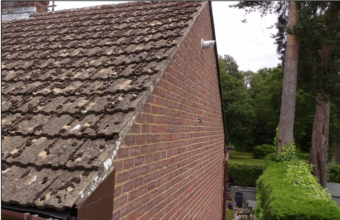
Figure 7. Example of sealed verges. 104 Reading Road, Finchampstead. 10.06.25
