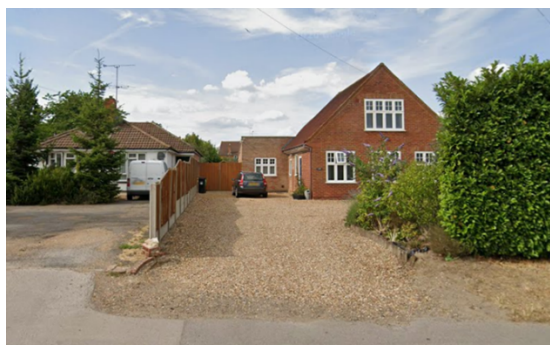
Figure 4 Google Street view Image of no's 117 and 119 Headley Road
