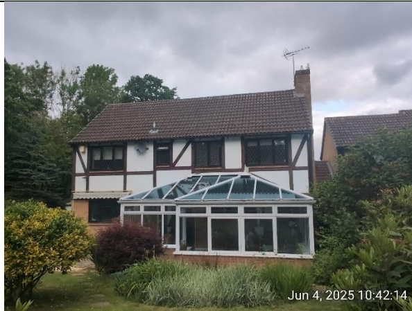
Figure 5: B1 southern elevation and conservatory
