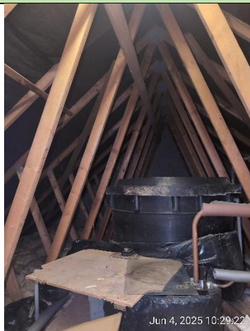
Figure 7: loft interior of B1
