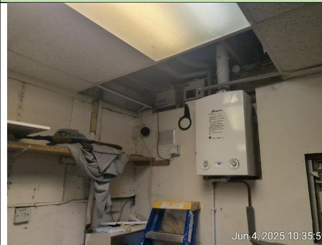
Figure 8: garage interior of B1
