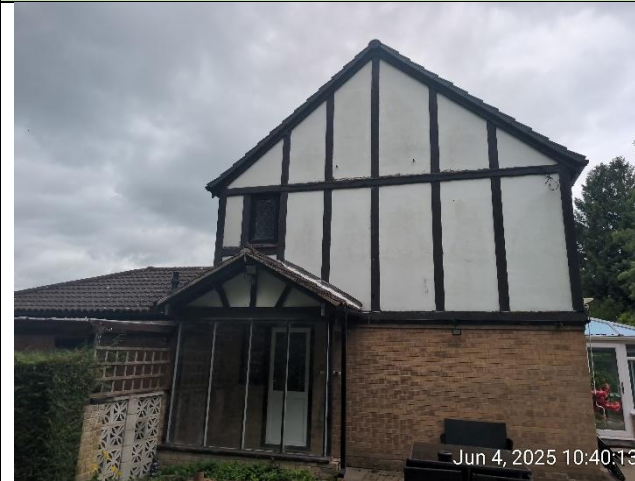
Figure 6: B1 western gable end
