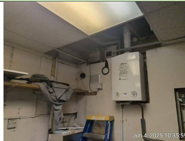
Figure 8: garage interior of B1
