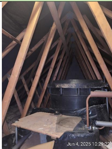
Figure 7: loft interior of B1
