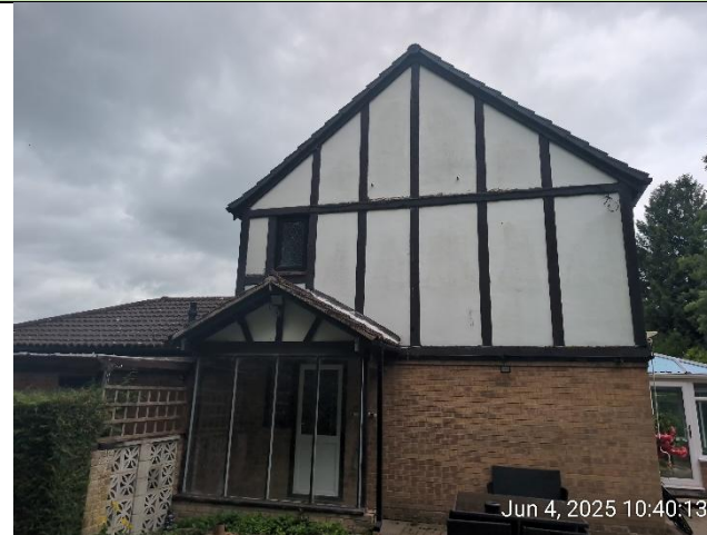
Figure 6: B1 western gable end
