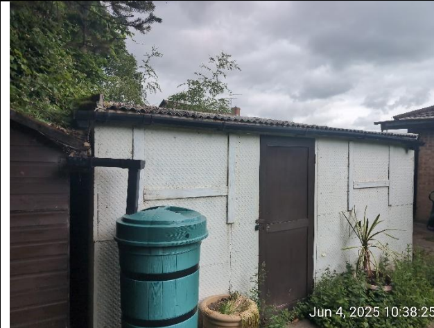
Figure 10: B2 view from south
