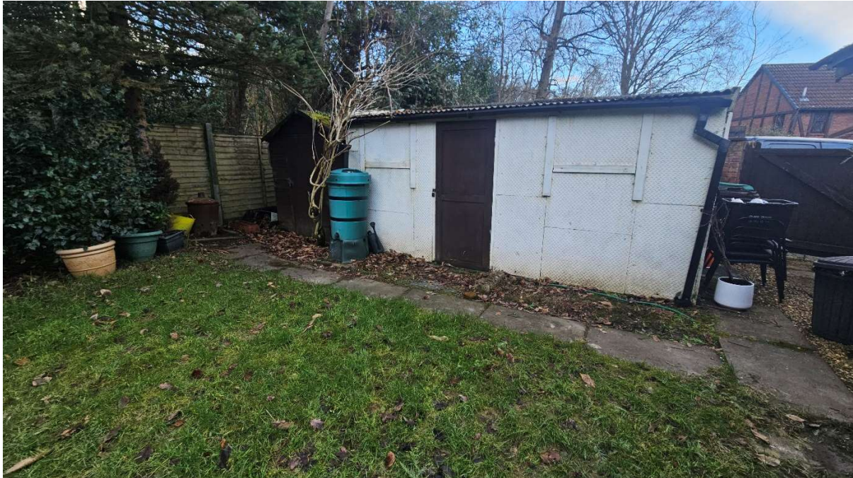
Fig. 4. Existing garage and shed looking north from the rear garden
