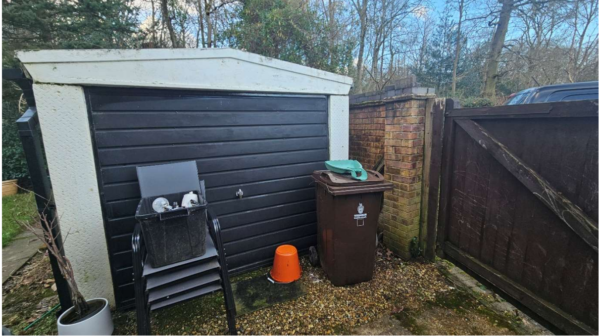
Fig. 5. Existing garage, garden wall and gate
