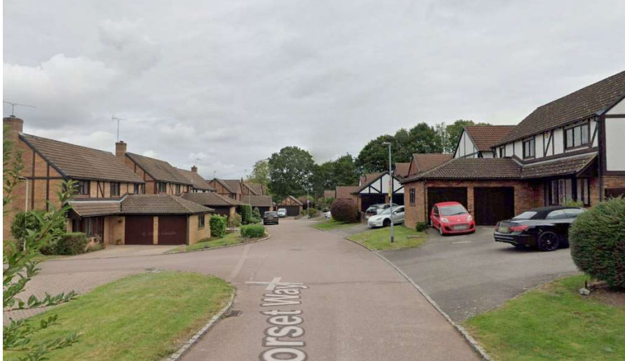
Fig 2. Frontage throughout the housing development have garages on the frontages of plots. Looking east along Dorset Way from outside No 65.
