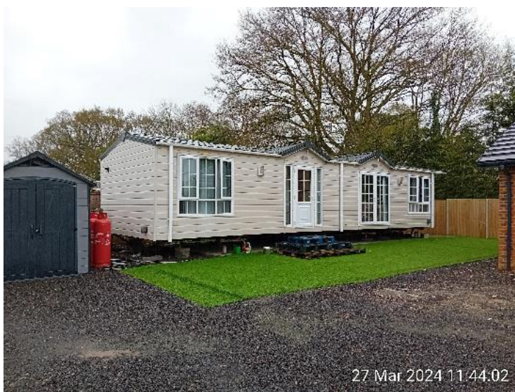
Figure 4: Front elevation of B2
