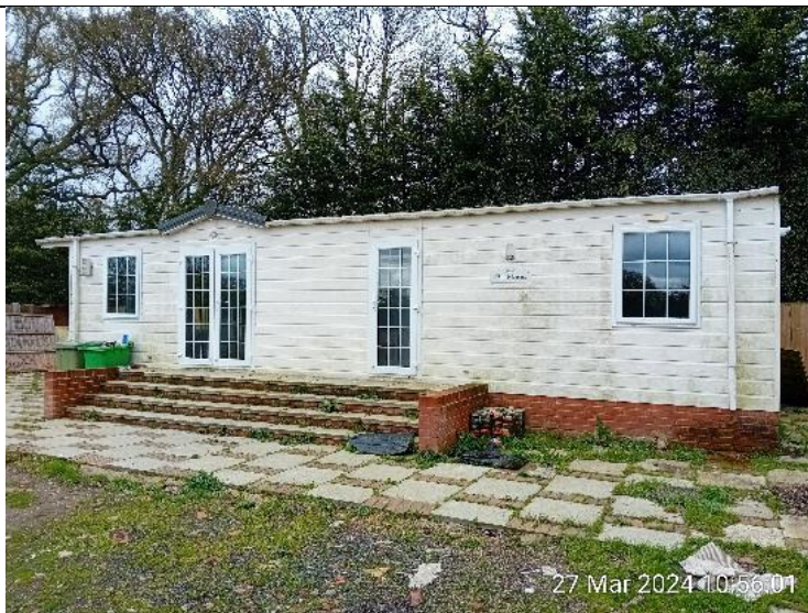
Figure 3: Front elevation of B1
