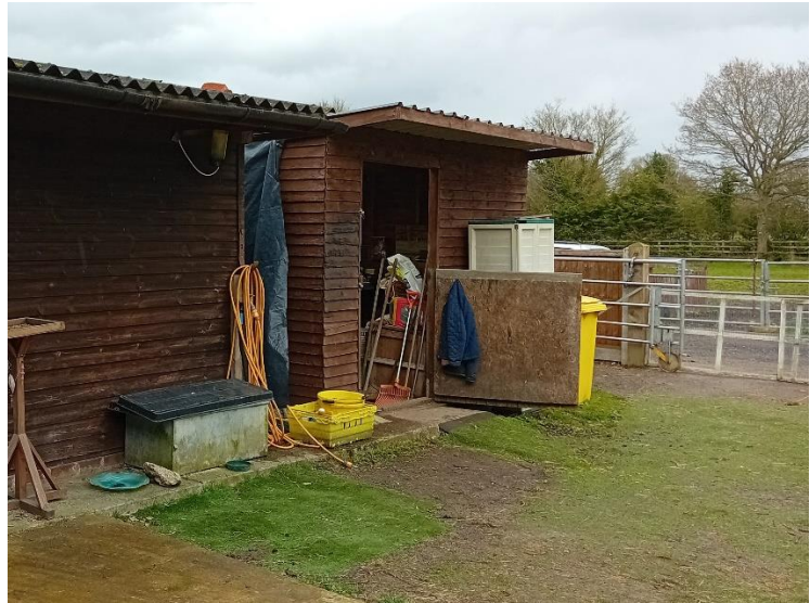
Figure 11: B7, located adjacent to B5
