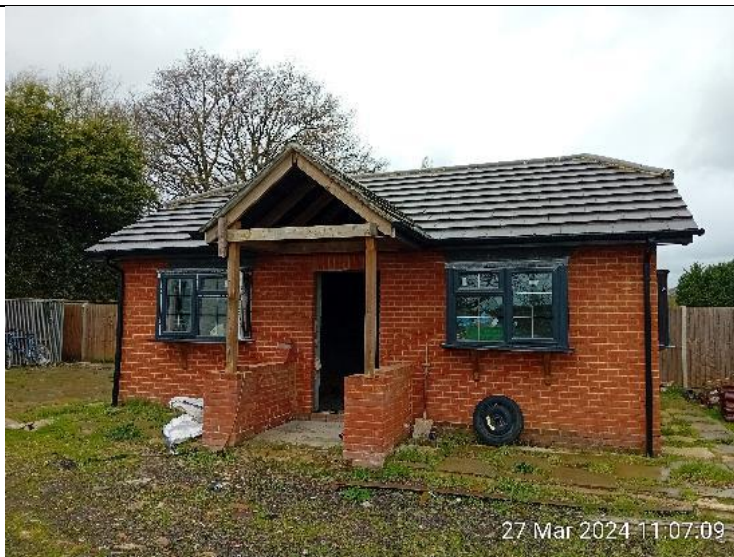
Figure 5: Exterior of B3 & B4.
