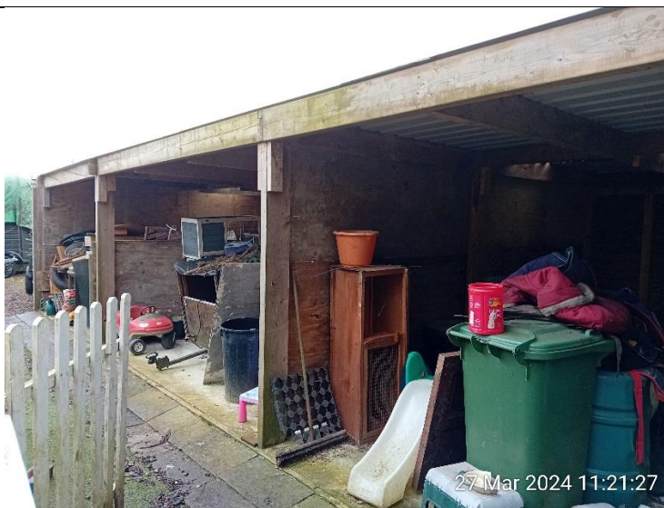
Figure 9: Lean to on the rear of B5
