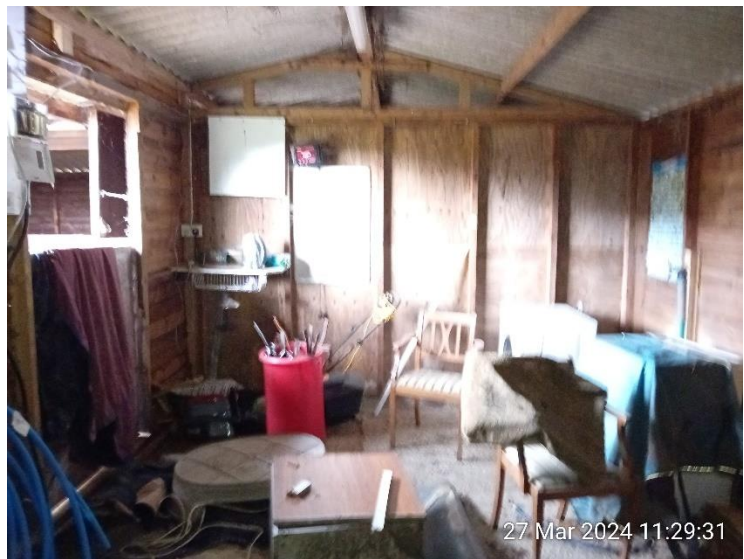
Figure 8: Example interior of B5
