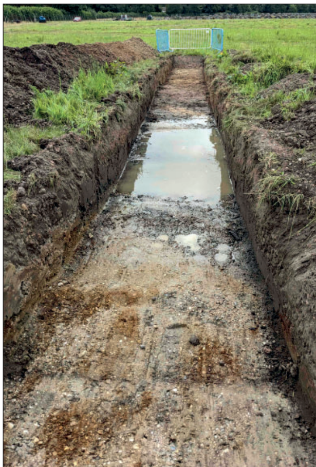
Figure 23: View of Trench 29 from north-west showing water ingress
