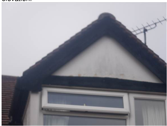
Photograph 10. Timbers tight on the rear dormer window.
