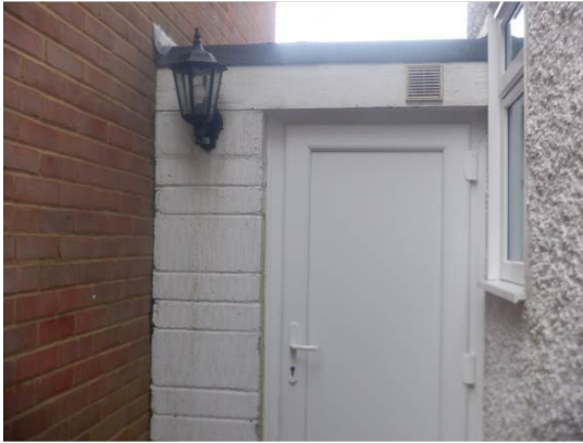
Photograph 11. Tight roof on the rear of the garage.
