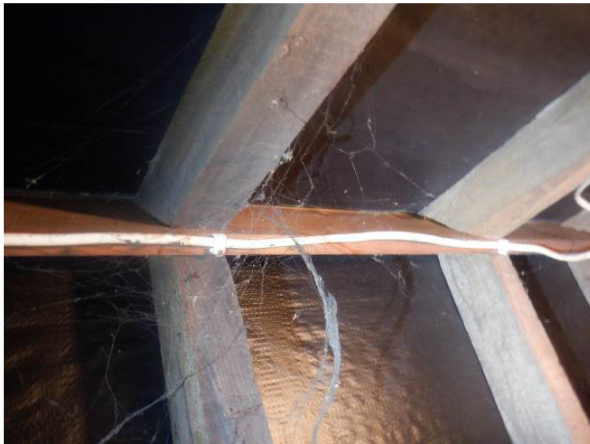
Photograph 12. Roof lined with a plastic style roofing lining.
