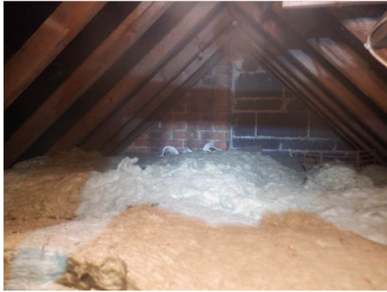
Photograph 14. Boarded floor covered with fibreglass,
