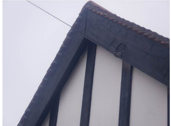
Photograph 6. Verge mortar intact on the front north western side elevation.
