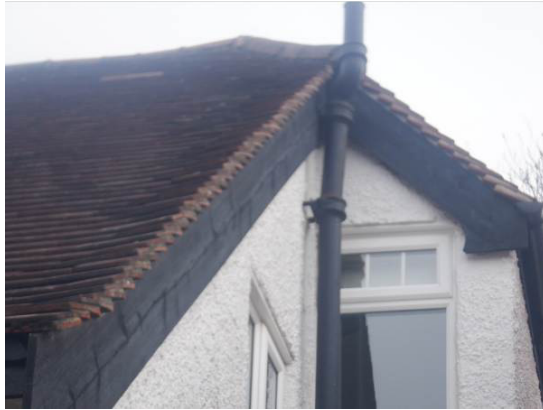
Photograph 5. Verge mortar intact on the south western side elevation.
