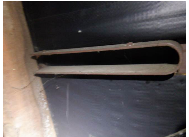
Photograph 13. Vents present in the roof.
