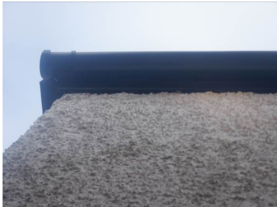
Photograph 7. Gaps along the fascias and rendered wall.
