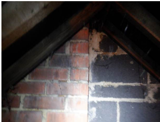
Photograph 16. Block work party wall with brick work chimney.
