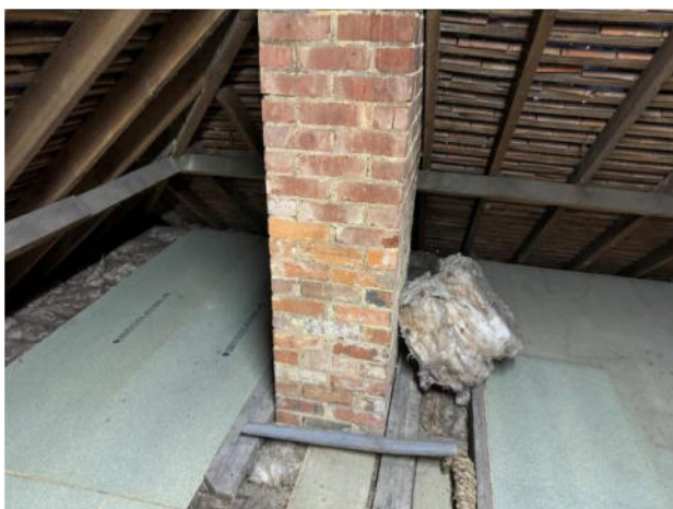
Photograph 5. The loft space of the building.
