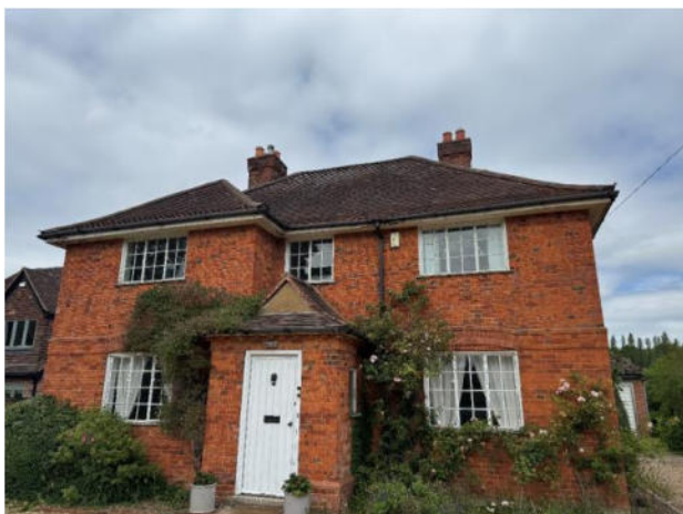
Photograph 1. The building viewed from the south.
