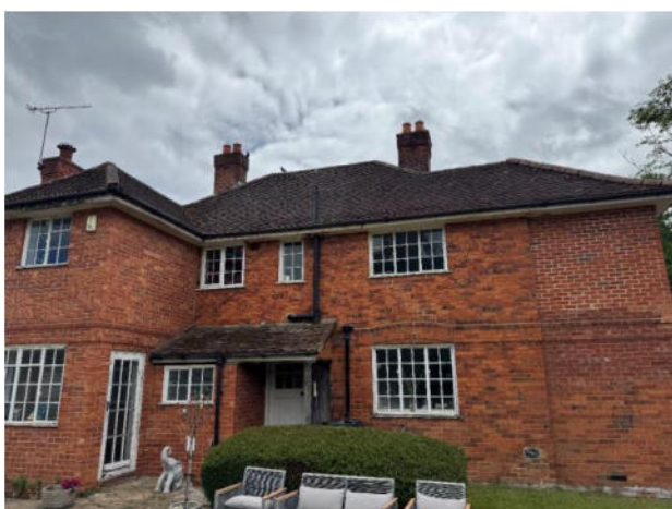
Photograph 3. The building viewed from the north.
