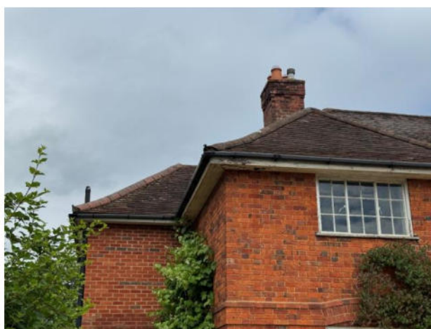
Photograph 4. The building viewed from the south-west.
