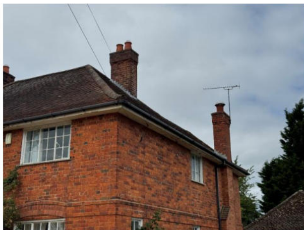
Photograph 2. The building viewed from the south-east.
