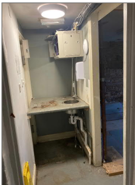
View of return wall at LHS of bar
