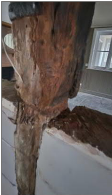
View of cut away timber post
