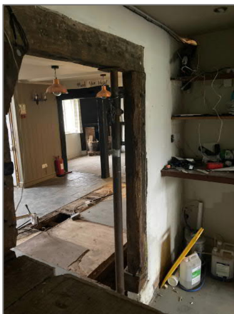
View of return wall at RHS of bar
