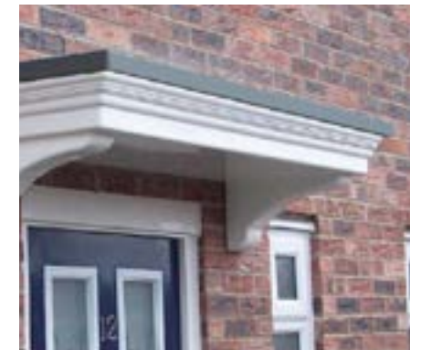
Flat roof porches
