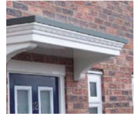
Flat roof porches
