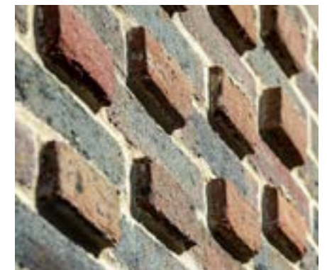
Protruding detailing forms
