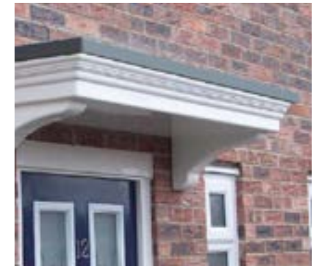
Flat roof porches
