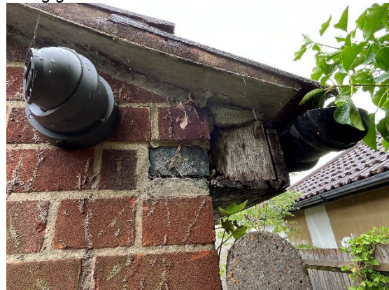
Photograph 14. Superficial decay at the end of the soffit on the western side of the pitched roof.
