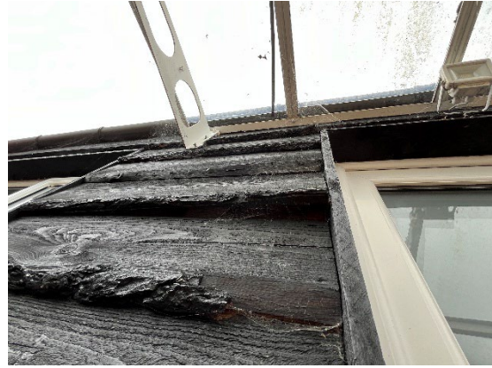
Photograph 16. Timber cladding at the southern end of the office building with slight gaps between boards.
