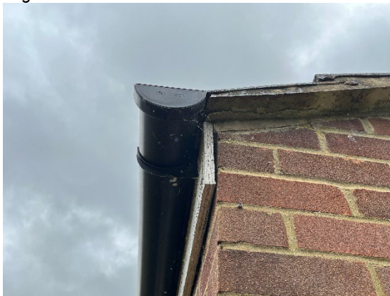
Photograph 13. Slightly raised barge board at north eastern corner.
