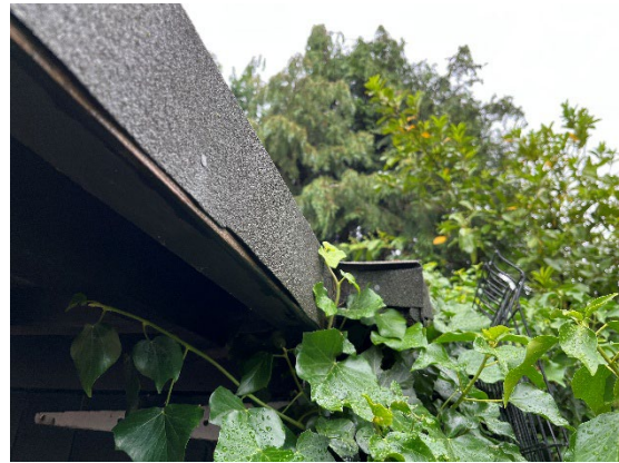
Photograph 18. The tightly fitted bitumen felt roof.
