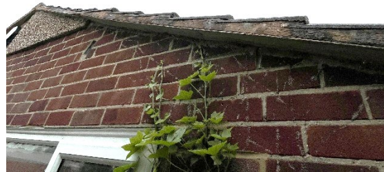
Photograph 12. Intact mortar and render at north facing gable end.
