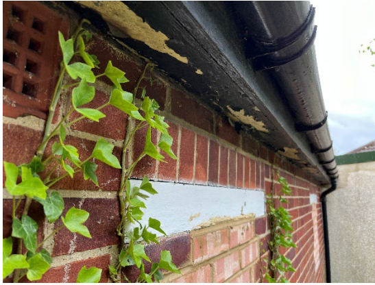
Photograph 15. Tightly fitted barge boards on western side of the northern section of the building.
