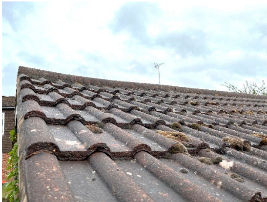
Photograph .11. Tightly fitted concrete roof tiles ad ridges.
