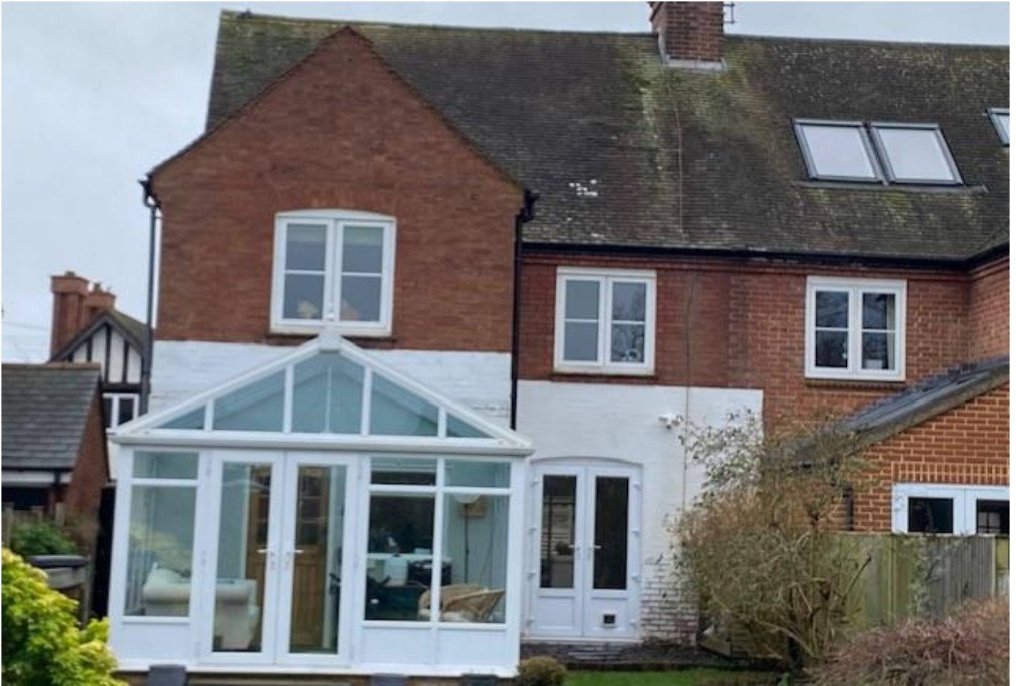
Photograph 2 Rear Elevation 40 Sturges Road Wokingham.
