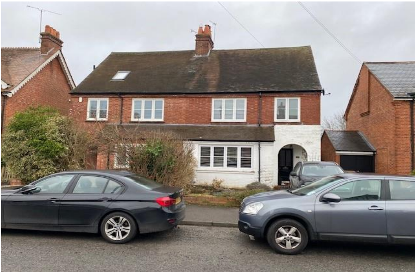
Photograph 1 Front Elevation 40 Sturges Road Wokingham (House with white painted brick at GF level)
