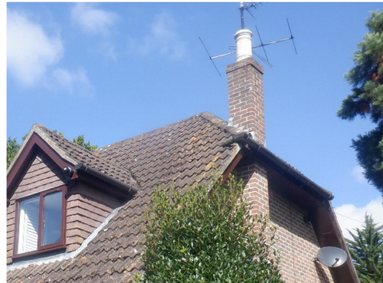
Photograph 4. Intact ridge, hip and verge mortar (rear elevation)
