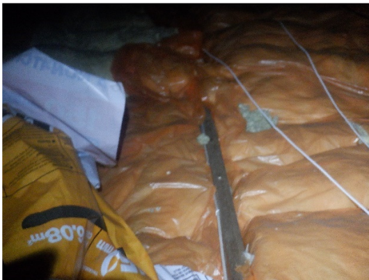
Photograph 16. Internal view of the roof void with fibreglass insulation in the northern section.
