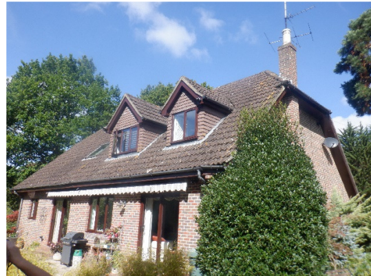
Photograph 2. Side and rear of house viewed from southwest.
