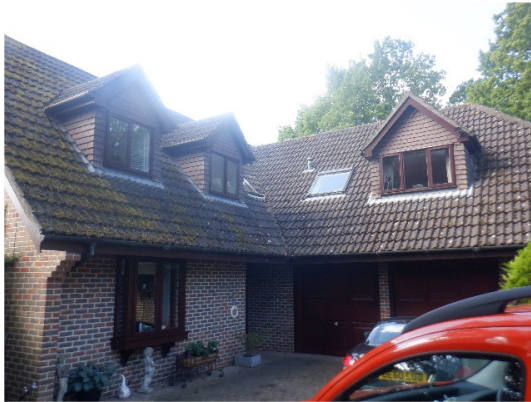
Photograph 1. Front of house viewed from northeast.
