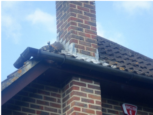
Photograph 7. Tight lead flashing against eastern chimney (eastern elevation).
