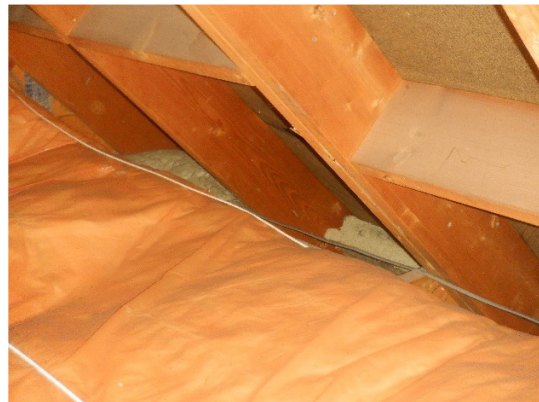
Photograph 17. Eaves filled with insulation boards in places (roof void).
