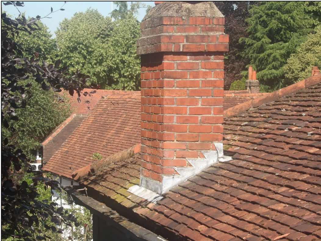
Figure 8. Example sealed lead flashing. Brook House, Hight Street, Sonning. 25.06.24
