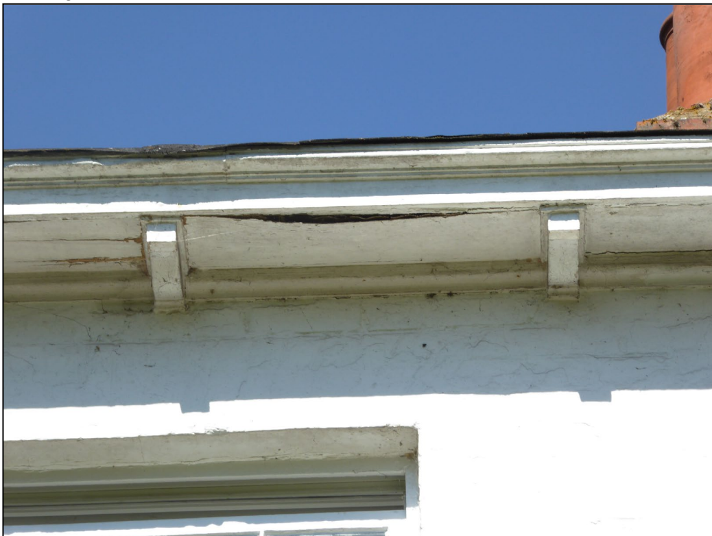
Figure 10. Split section of flat eaves on rear elevation. Brook House, Hight Street, Sonning. 25.06.24
