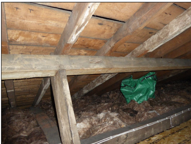
Figure 12. Example warped timber sarking. Brook House, Hight Street, Sonning. 25.06.24
