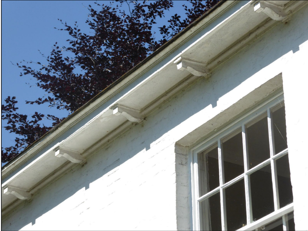
Figure 9. Example sealed flat eaves and brackets. Brook House, Hight Street, Sonning. 25.06.24
