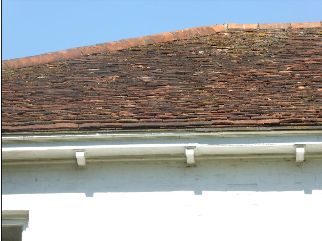
Figure 4. Examples of spalling/delaminated roof tiles. Brook House, Hight Street, Sonning. 25.06.24
