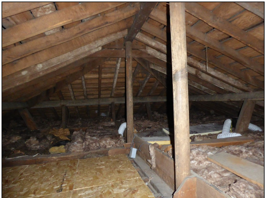
Figure 12. Example warped timber sarking. Brook House, Hight Street, Sonning. 25.06.24
