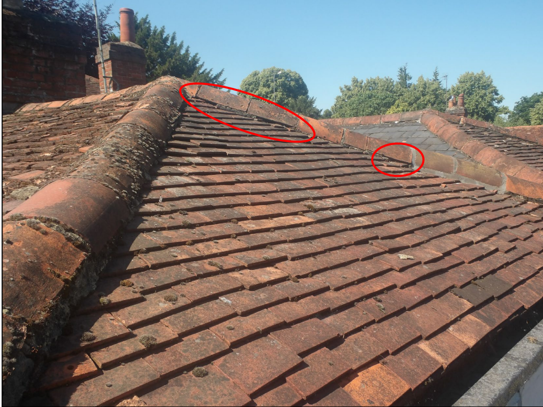
Figure 7. Example missing mortar from hip tiles. Brook House, Hight Street, Sonning. 25.06.24
