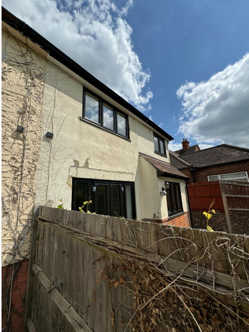
Rear Elevation – towards no.108
