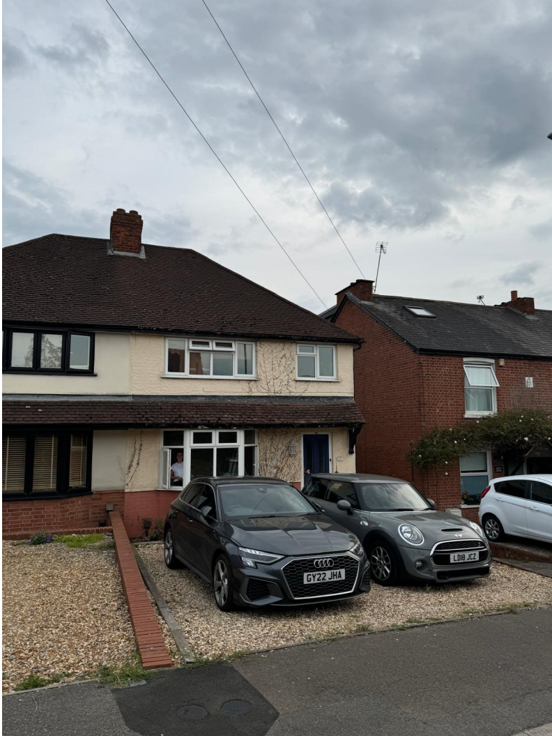
Front Elevation – general view
