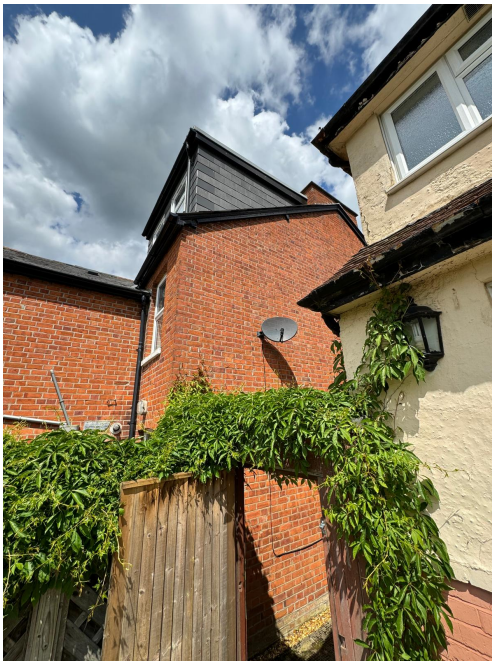
Rear Elevation – towards no.112
