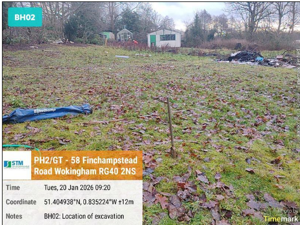
Image showing the location of BH02
