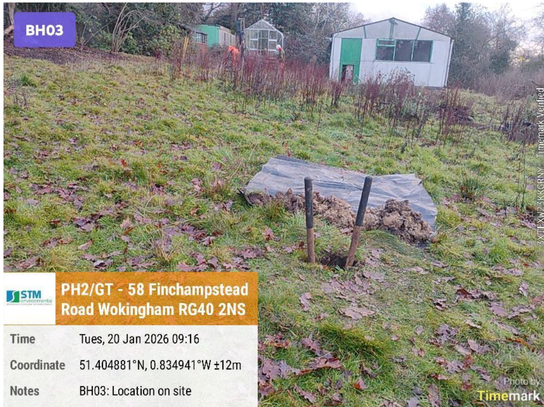
Image showing the location of BH03
