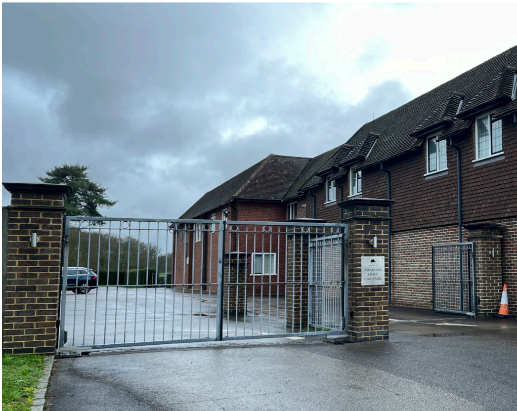
1 Figure 15. Existing Gates to Members Car Park
