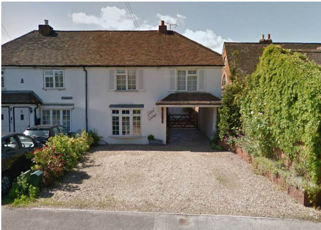
North Facing Front Elevation of 1 Talbot Cottage, Forest Road, Binfield, RG40 5SG
