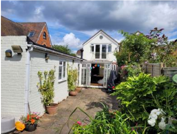
Existing conservatory to be demolished
