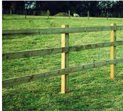
POST AND RAIL FENCING
