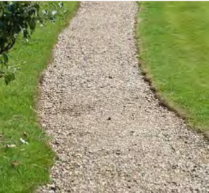
SELF-BINDING GRAVEL FOOTPATH
