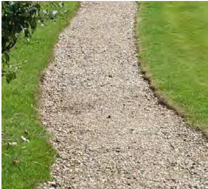
SELF-BINDING GRAVEL FOOTPATH
