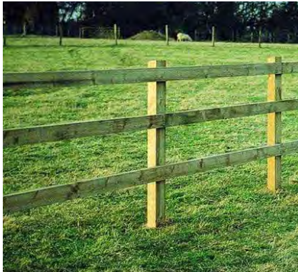
POST AND RAIL FENCING
