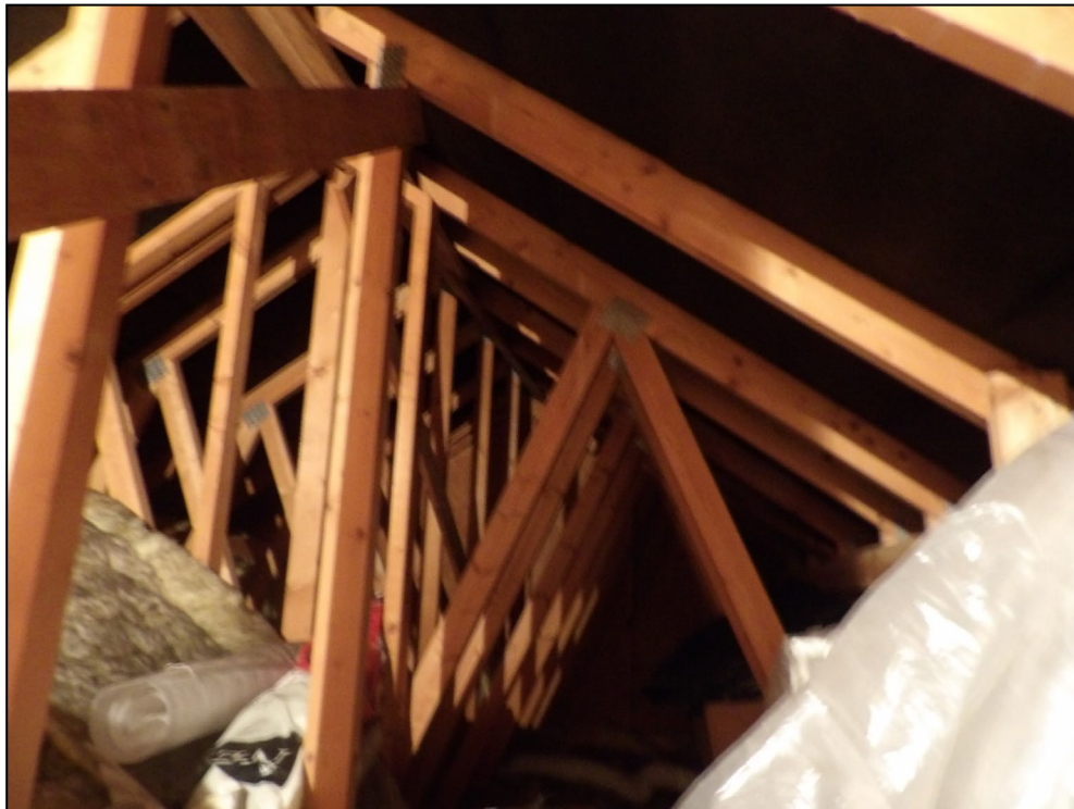
Figure 9. Example of loft space and bitumen felt. 98 Broad Hinton, Twyford. 03.12.24
