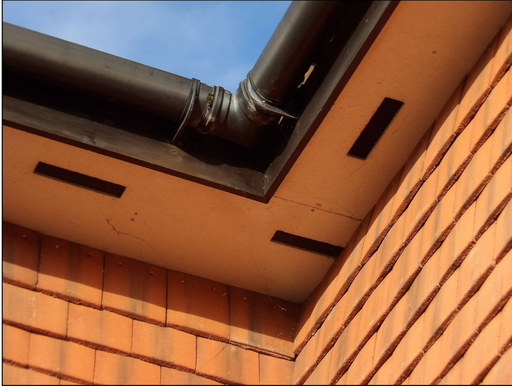
Figure 7. Example of soffits/fascias and ventilation holes. 98 Broad Hinton, Twyford. 03.12.24
