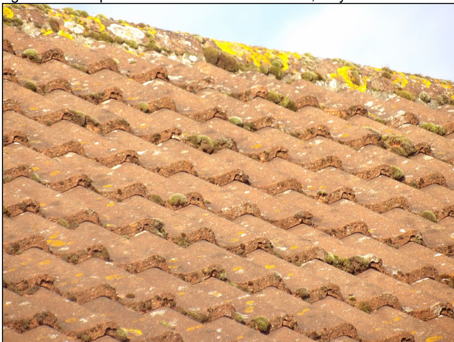
Figure 4. Example of roof tiles. 98 Broad Hinton, Twyford. 03.12.24
