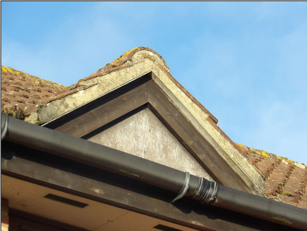
Figure 6. Dormer on front elevation. 98 Broad Hinton, Twyford. 03.12.24
