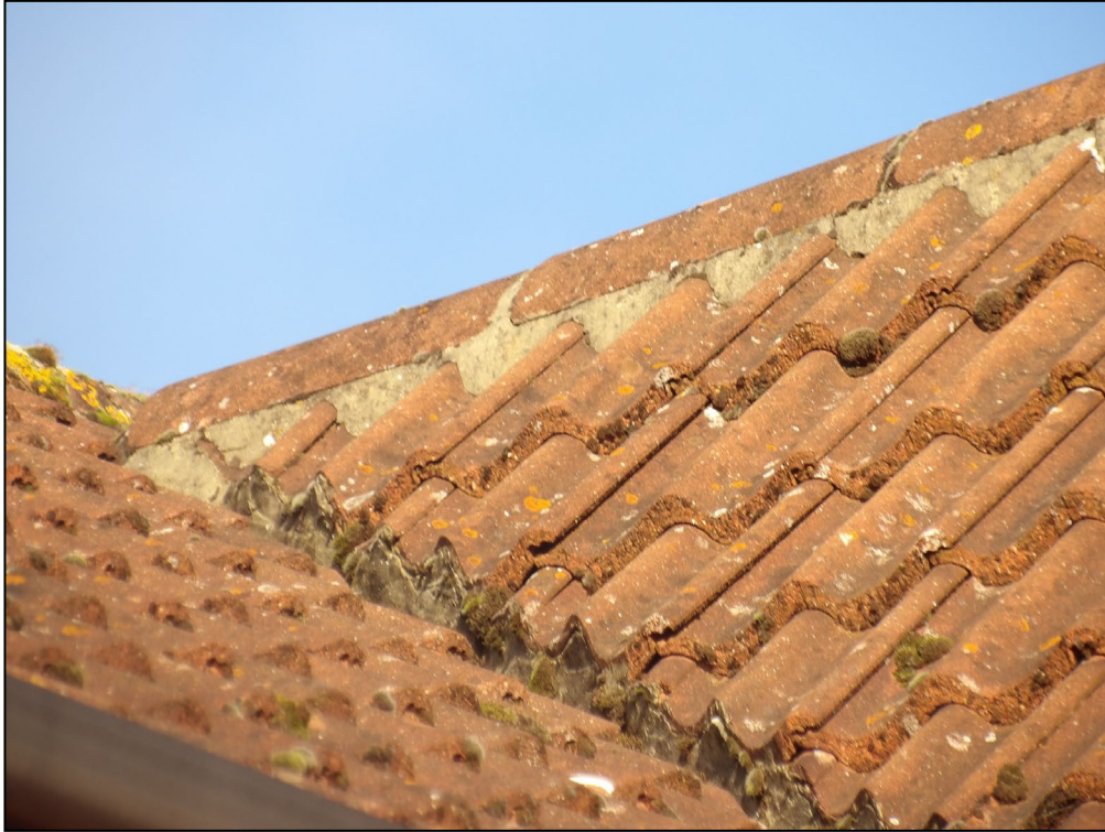
Figure 5. Example of ridge tiles. 98 Broad Hinton, Twyford. 03.12.24
