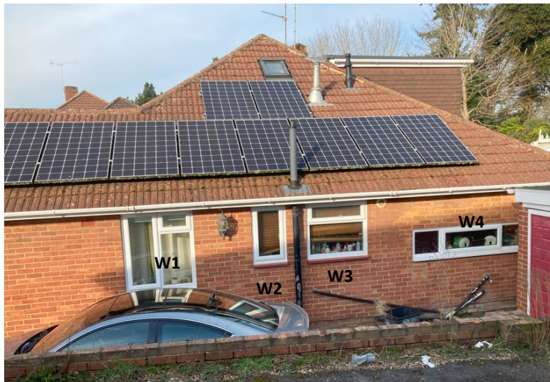
Flank Wall of No.33
