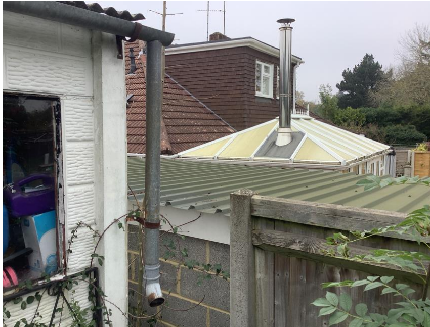
View of Rear of No.33 (taken from rear of garage of host property)
