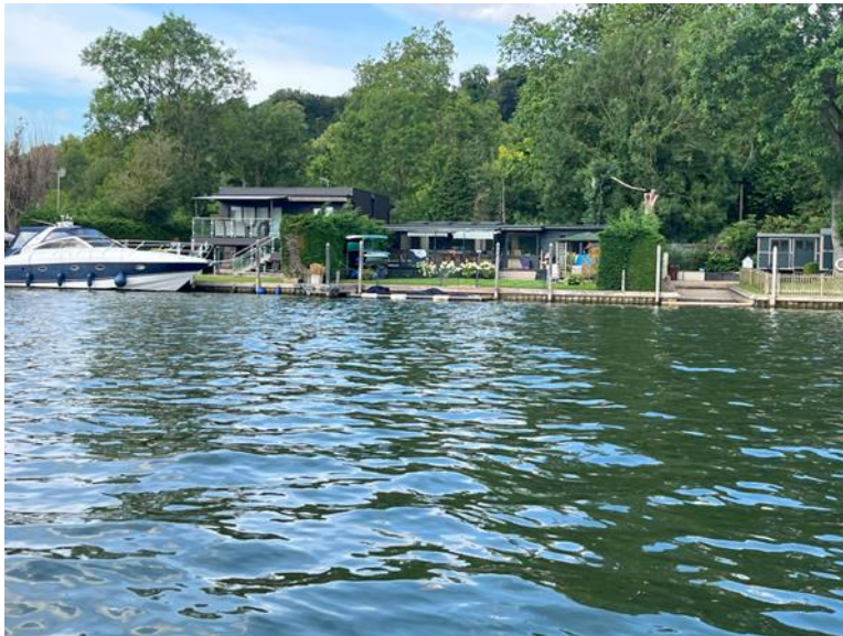
Photo 1 - Photo of the application site viewed from River Thames with 2 Riverside in the middle. To the right of the photograph is plot 3 with a higher dwelling with a flat roof. To the right of the photograph is plot 1 Riverside.
