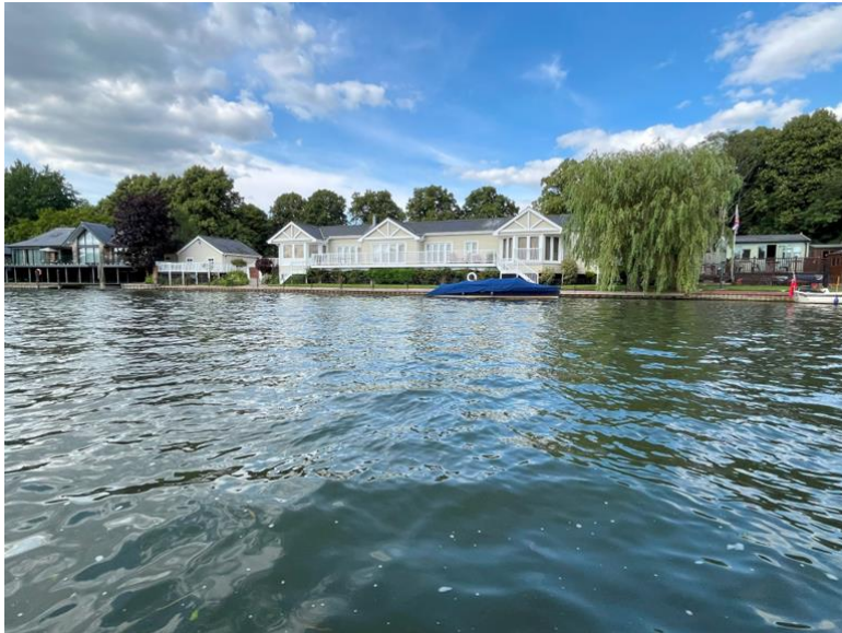
Photograph 4 – Pitch roof with 3 gable features facing the River at ‘The Landing’ sited to the north west of the application site viewed from the River Thames. To the left of the photograph is Kilgarran.
