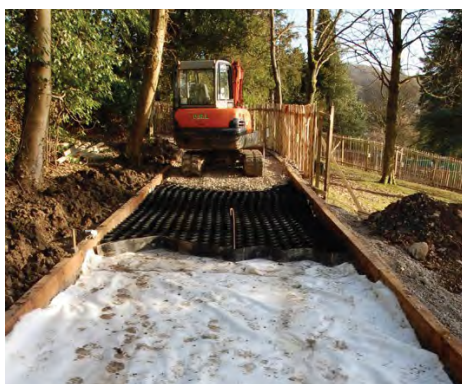
Fallbarrow Park, Windermere: CellWeb TRP® Installation
