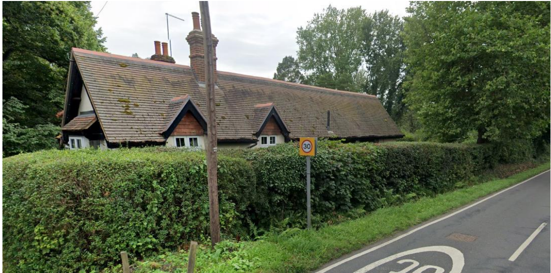
Property as viewed from Street
