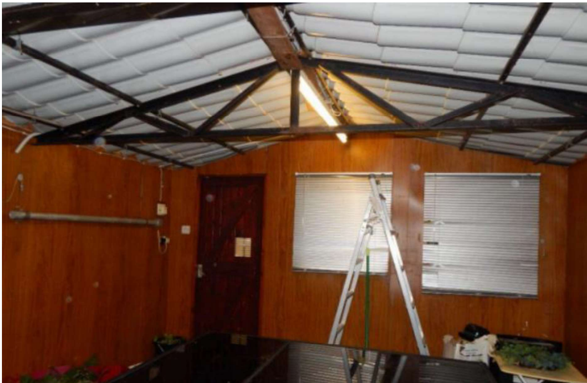
Image 12 – As above, internal views from below the fabricated roof coverings
