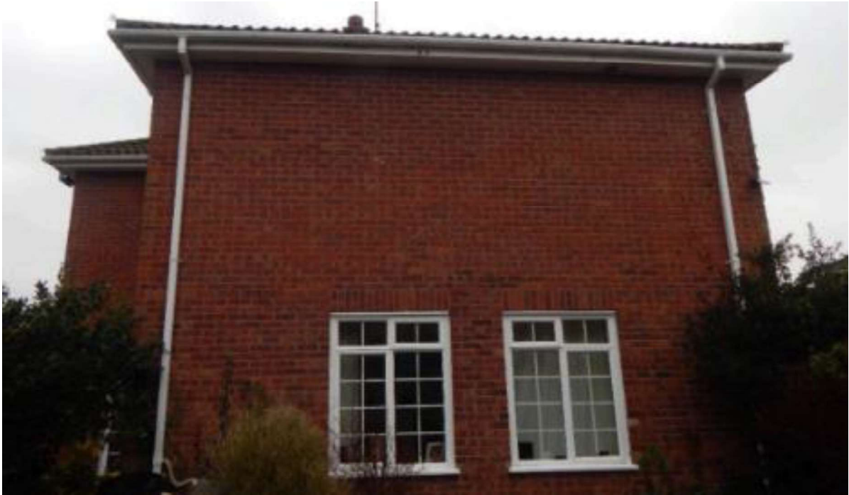
Image 3 – East facing elevation of the property
