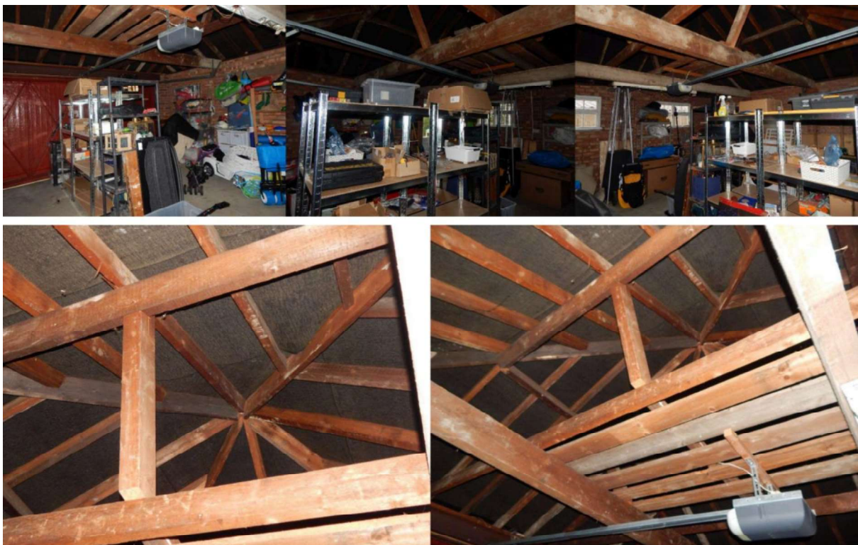
Image 10 – Internal view from within the detached garage
