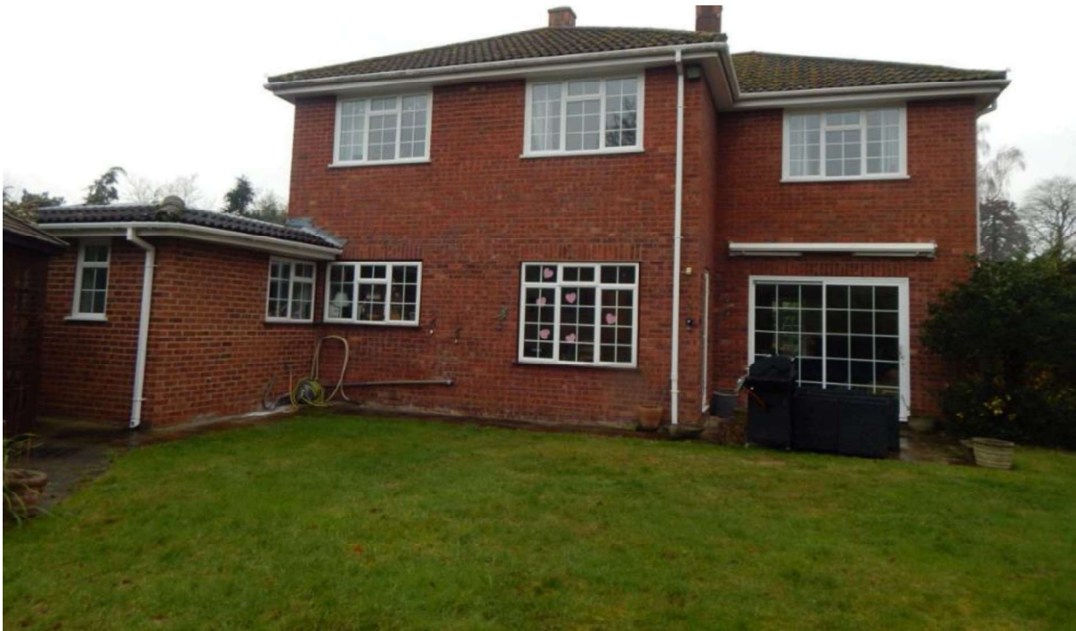
Image 2 – South facing elevation of the property
