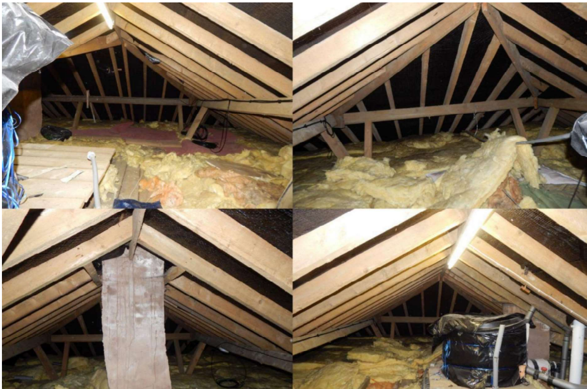
Image 7 – Internal views from within the main upper roof void spaces of the property
