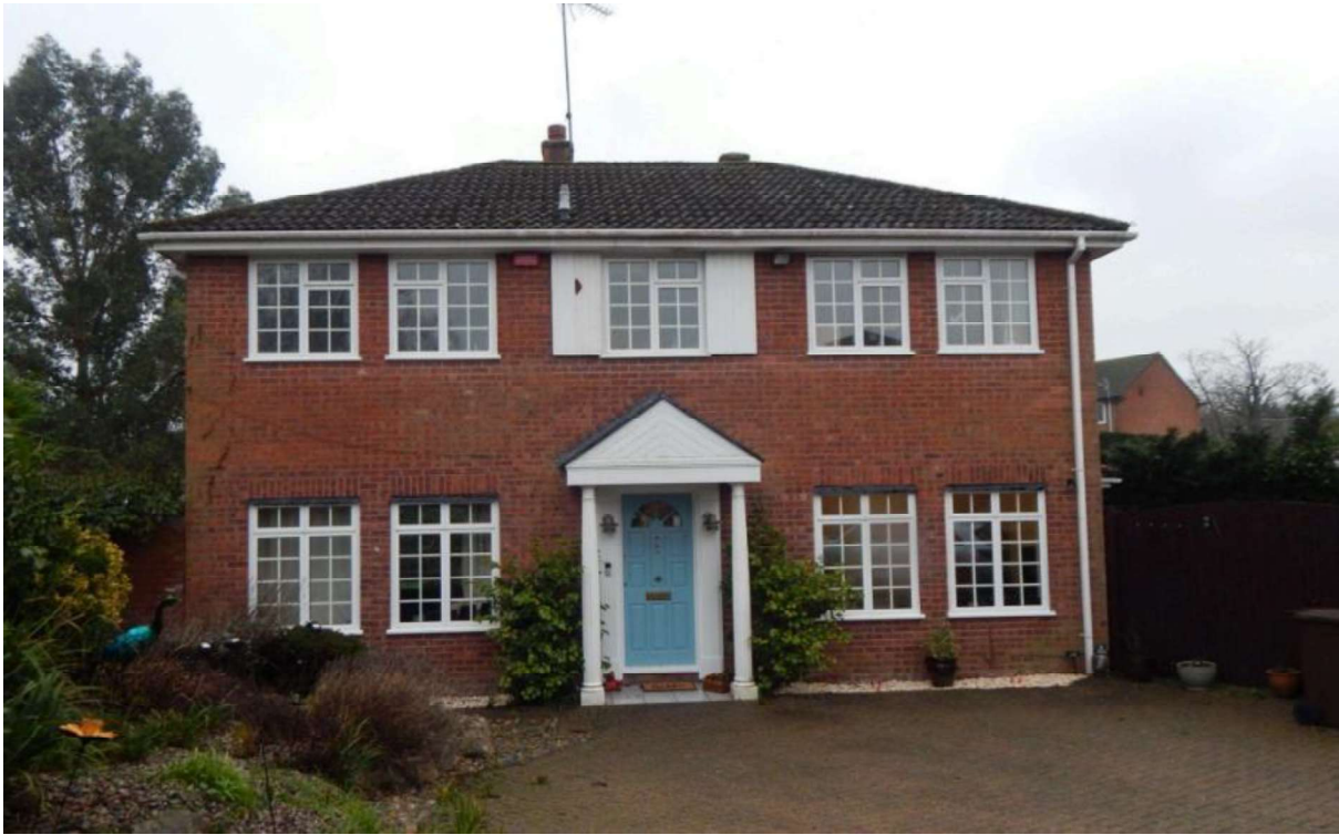
Image 1 – North facing elevation of the property
