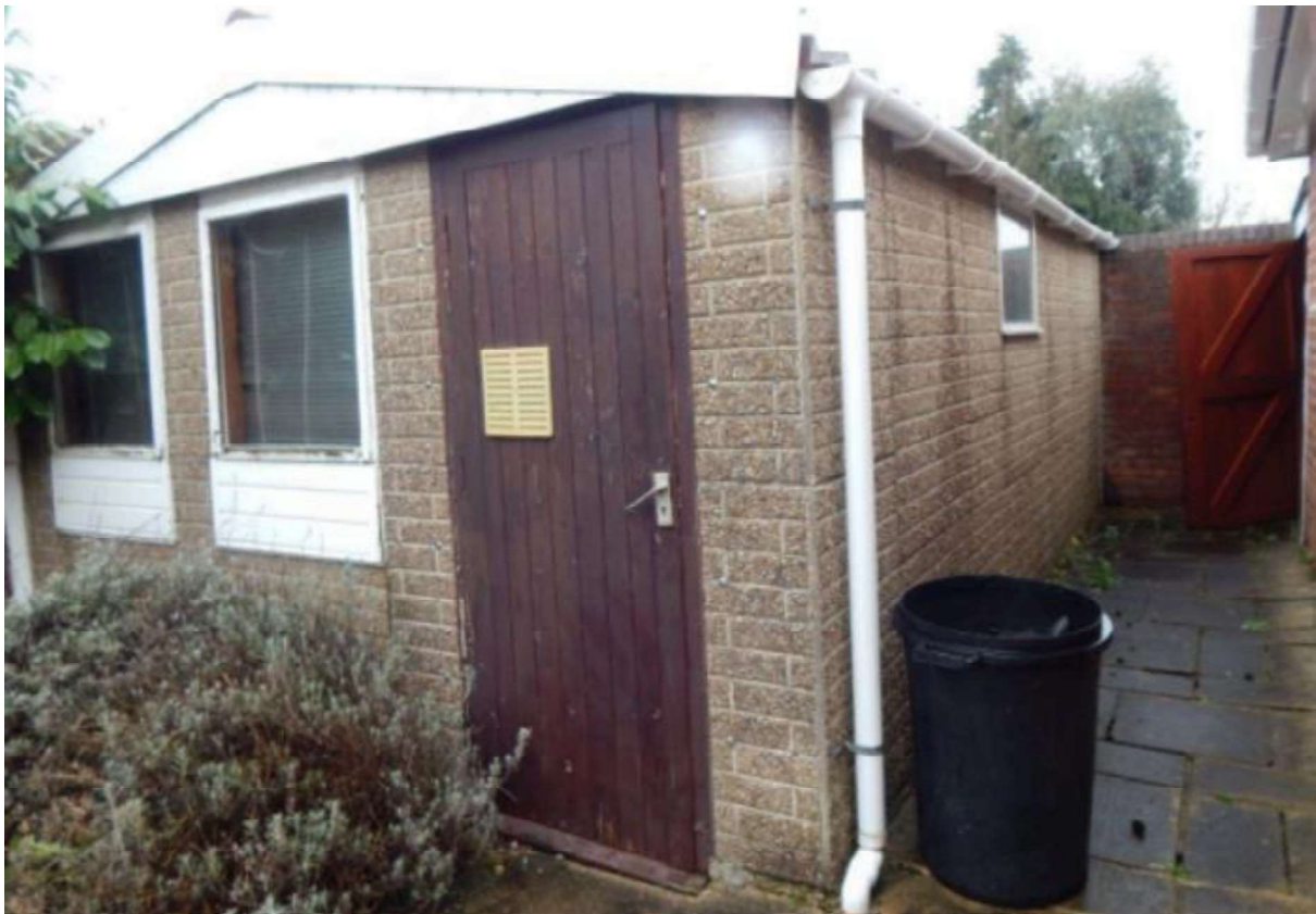
Image 11 – Outbuilding located to the side of the maid dwelling
