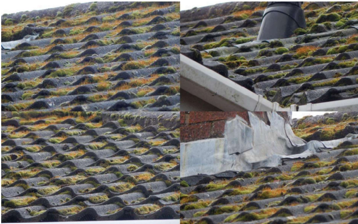
Image 5 – Close views of the tiled roof covering to show examples of condition
