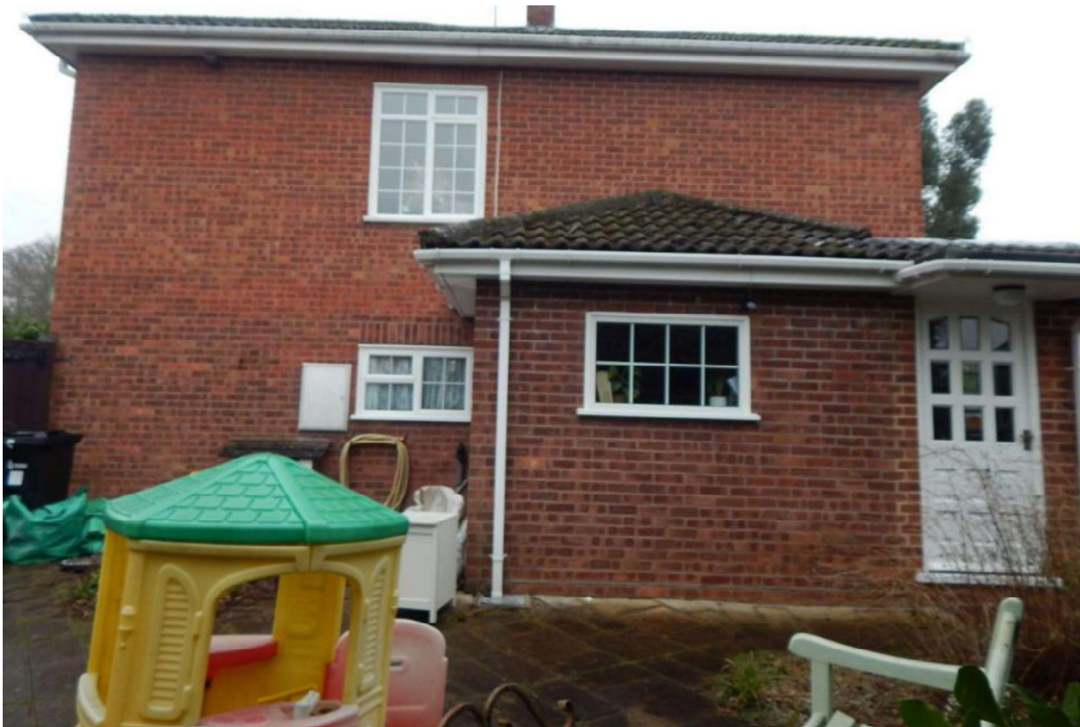
Image 4 – West facing elevation of the property
