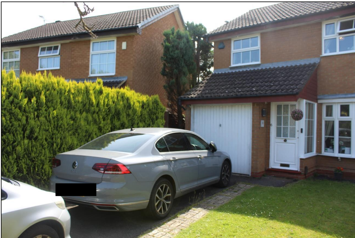
Photograph 1 – Front elevation as viewed from Vickers Close
