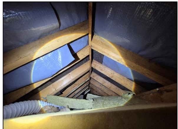
Photo 14: Main house loft void.
