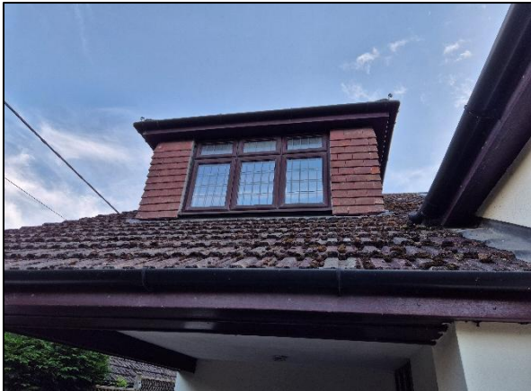
Photo 7: Dormer to be enlarged.
