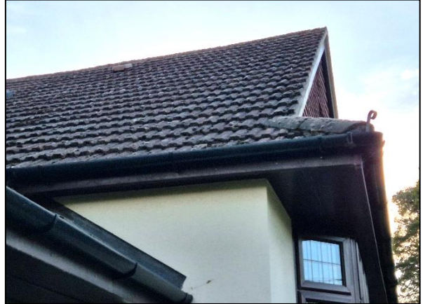
Photo 10: East facing roof slope.
