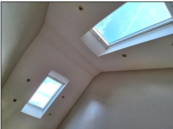
Photo 13: Interior of kitchen (no void).
