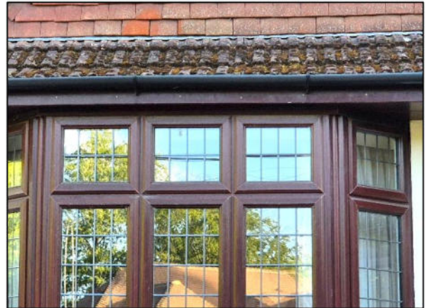
Photo 12: Small roof at front of house to be removed.
