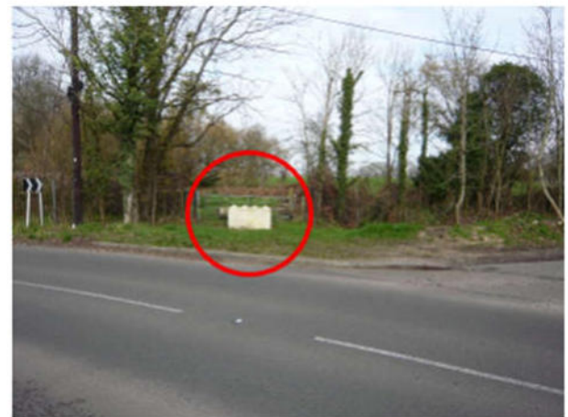
View looking north towards junction of proposed site access (ringed) / Wick Hill Lane.
