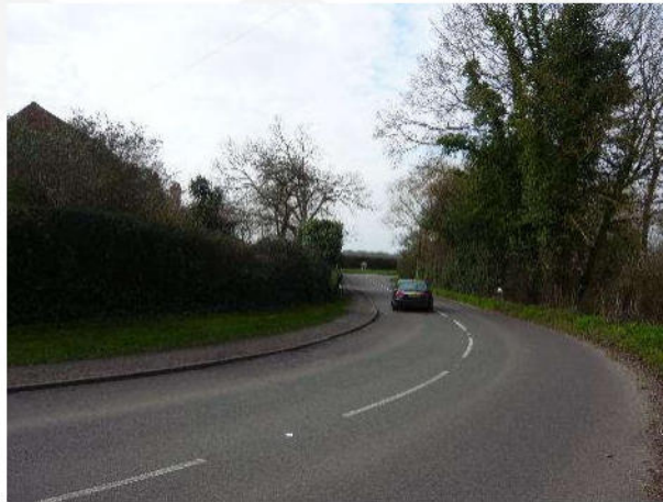
View of existing partially worn centre line markings along Jubilee Road.
