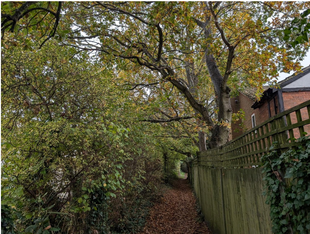
Figure 16: showing significant overhang across public footpath and into neighbouring properties 1
