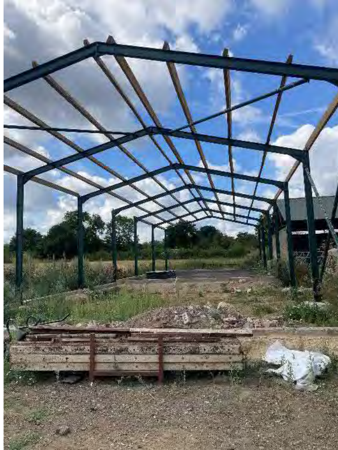
Photograph 11 – Construction of a fourth barn within Hambridge Farm (facing south)
