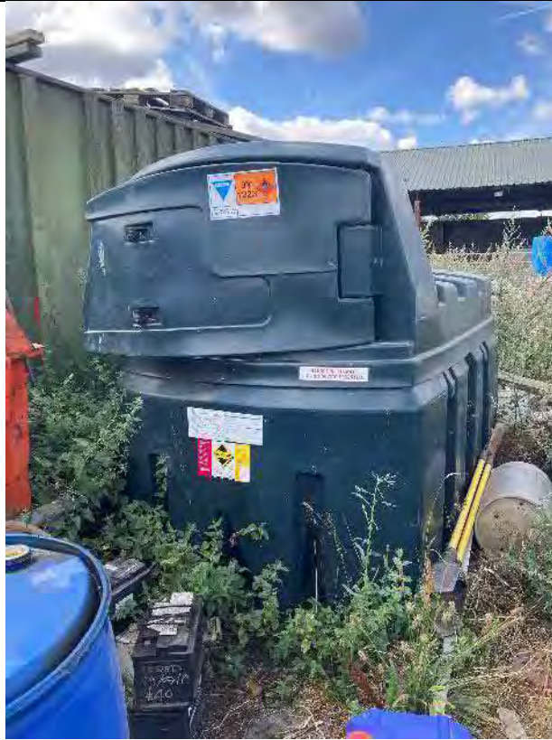
Photograph 17 – Tank 2 containing Kerosene located south of Barn 1 (facing north)
