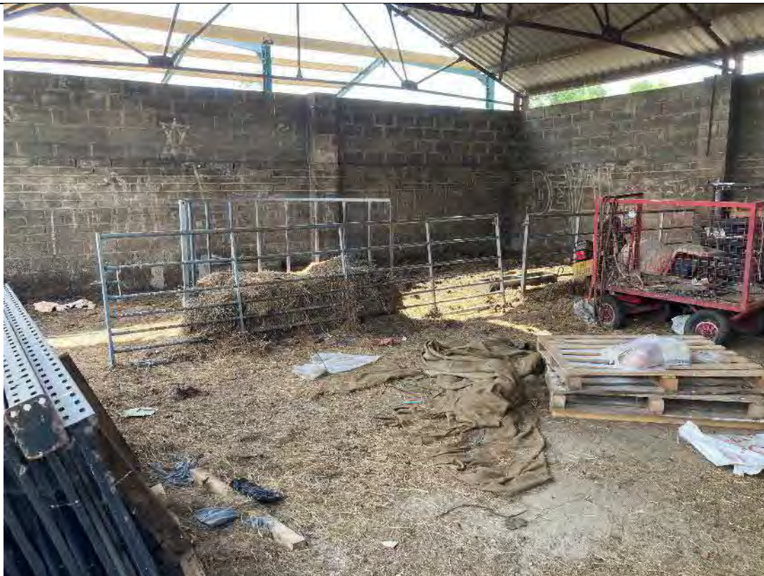
Photograph 8 – Internal access of Barn 1
