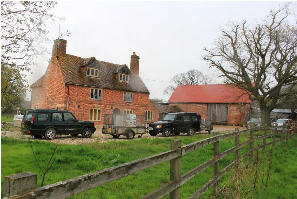
Image EDP A1.14: North facing view from the public footpath located immediately south of Britton's Farm. Image of Britton's Farmhouse on left side ( 1319141 ) and barn on right side ( 1118083 ), illustrates the immediate courtyard setting of the farm and the character and appearance of the front facing elevation to the farmhouse building.
