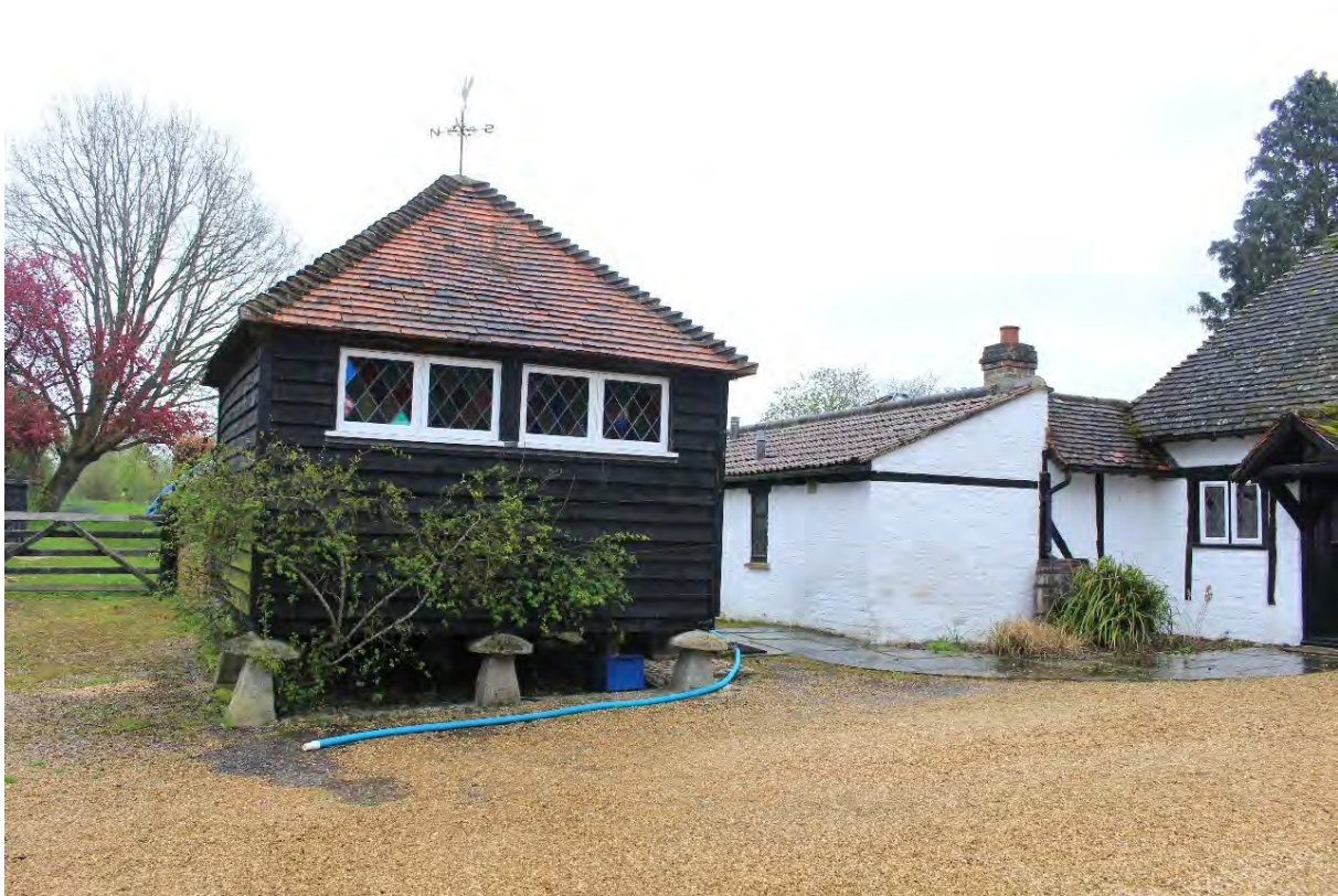
Image EDP A1.13: East facing view from within Pearce's Farm's farmyard. View of the listed granary ( 1135768 ) associated with the farm. The west corner of the modern indoor pool extension to Pearce's Farmhouse ( 1319115 ) is shown on the right-hand side of the image, in which the sympathetic design and appearance of the pool extension's perimeter is illustrated.
