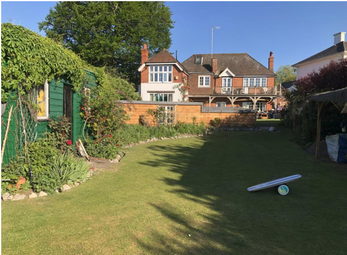
North West elevation of the former boathouse, now a single dwelling house.
