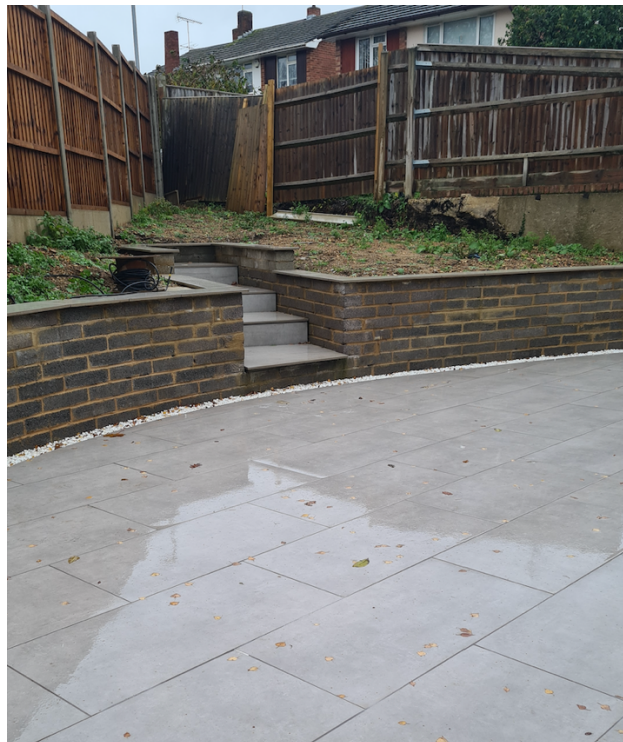
Figure 2 – Image showing hard landscaping to the rear garden
