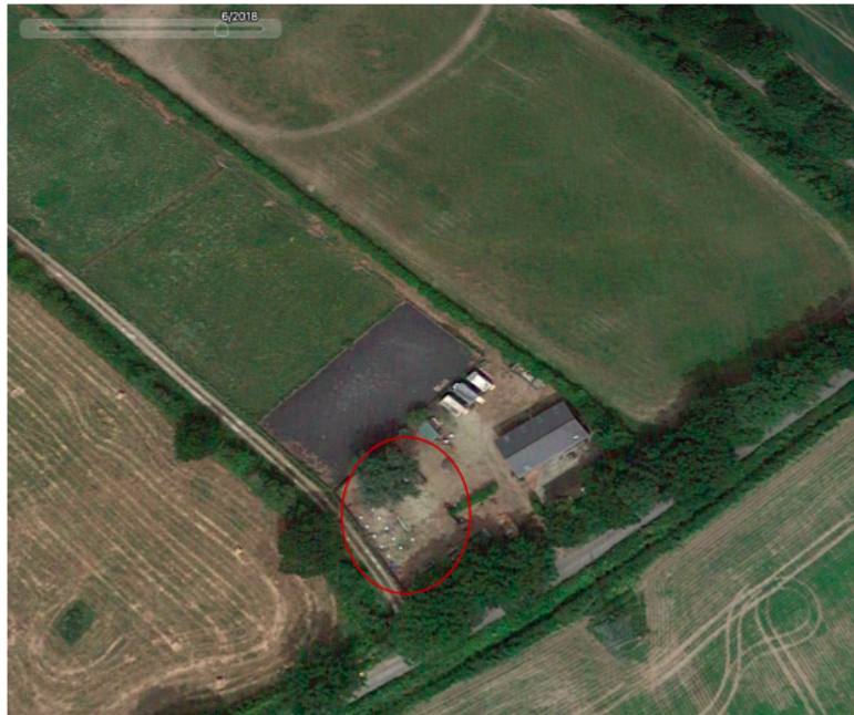
Figure 2: June 2018 Aerial Photograph
