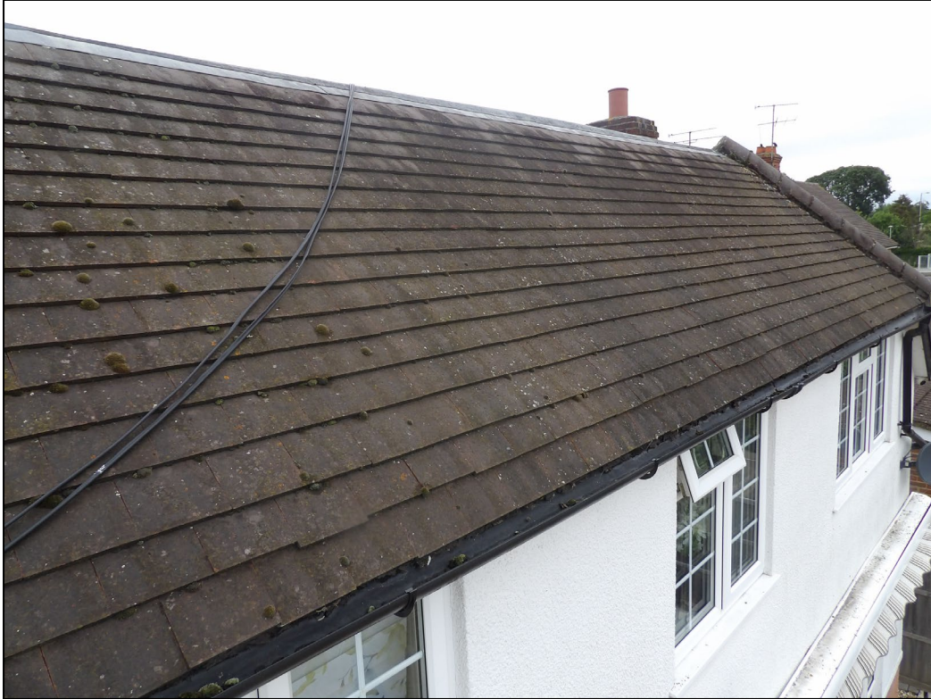
Figure 5. Example of composite tiles on rear extension. 98 Pitts Lane, Earley. 24.06.25
