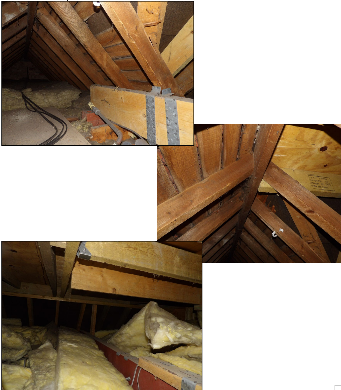
Figure 13. Example of loft space and timber sarking/plywood/bitumen felt lining. 98 Pitts Lane, Earley. 24.06.25
