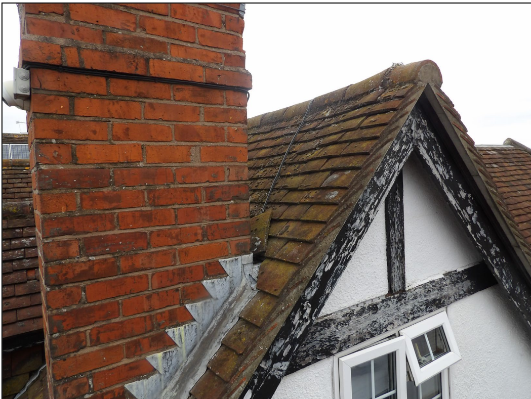
Figure 8. Example sealed verges. 98 Pitts Lane, Earley. 24.06.25
