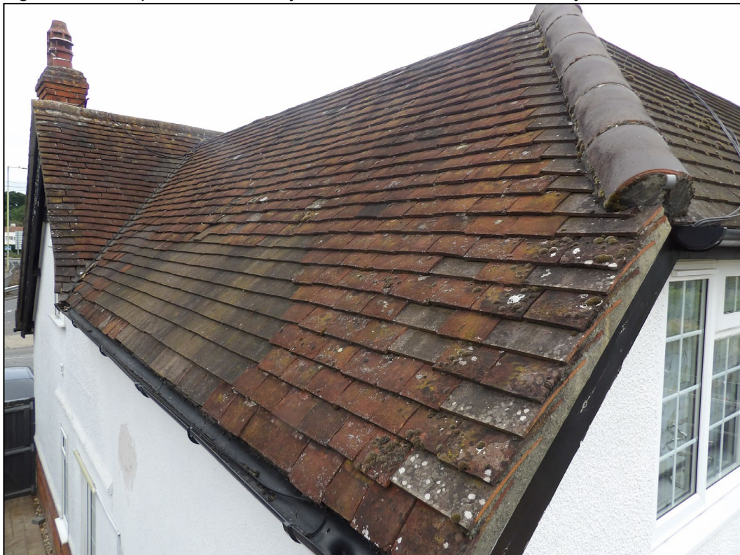
Figure 4. Example of sealed clay roof tiles. 98 Pitts Lane, Earley. 24.06.25
