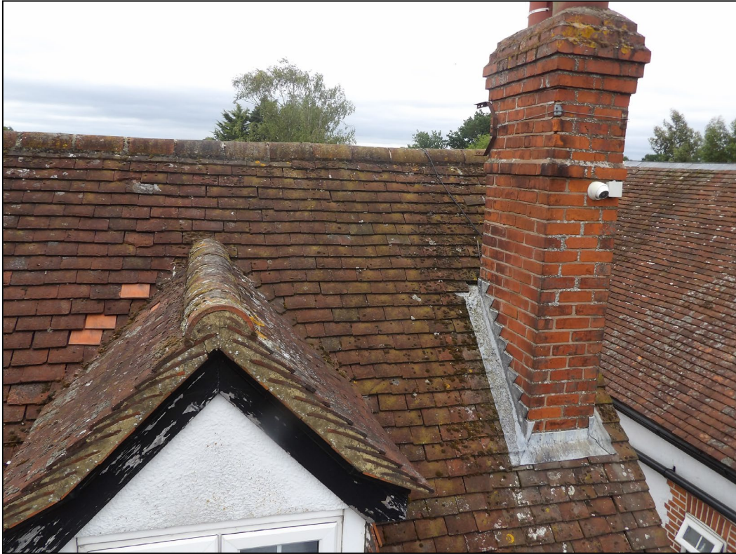
Figure 7. Example sealed ridge tiles and roof tiles on dormer and lead flashing. 98 Pitts Lane, Earley. 24.06.25
