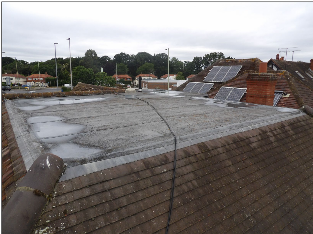
Figure 6. Example sealed bitumen felt on rear flat roof extension. 98 Pitts Lane, Earley. 24.06.25
