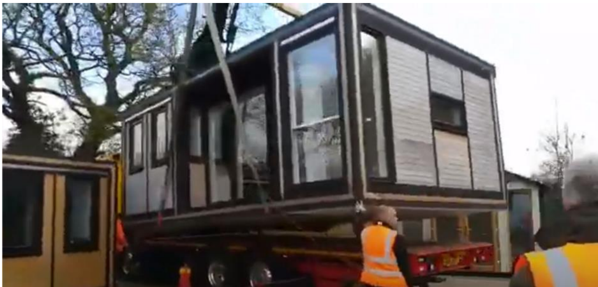
Figure 1 Removal of annexe by truck/hoist
