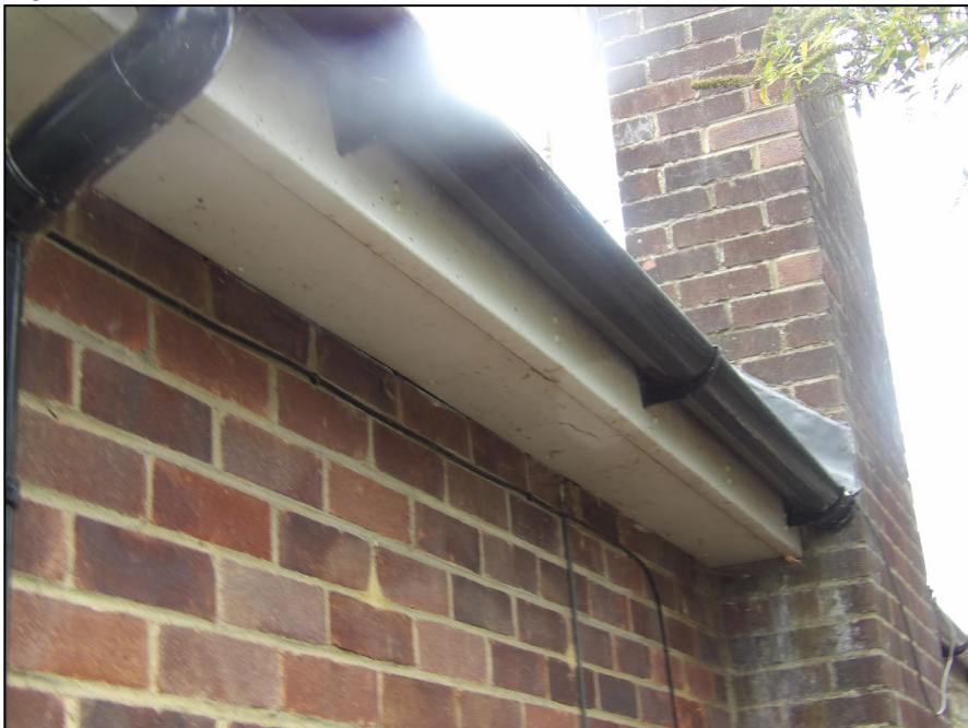
Figure 8. Example sealed soffits and fascias. 3 Garde Road, Sonning. 02.09.25
