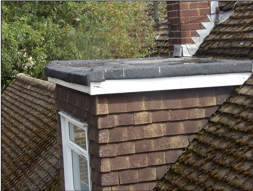
Figure 9. Bitumen covering dormer roof. 3 Garde Road, Sonning. 02.09.25
