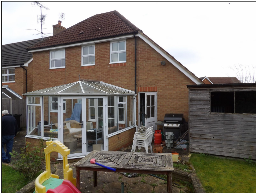
Figure 8. Rear view of property and conservatory. 196 Hurricane Way, Woodley. 17.03.26
