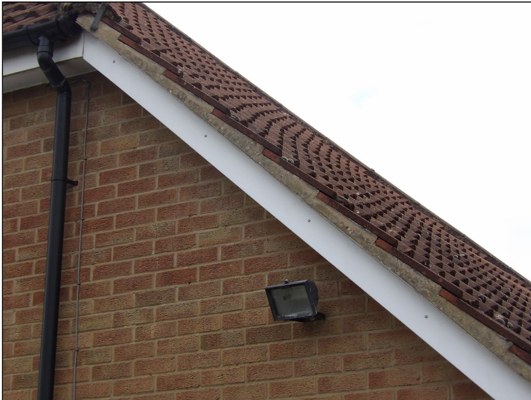
Figure 5. Example sealed verges. 196 Hurricane Way, Woodley. 17.03.26
