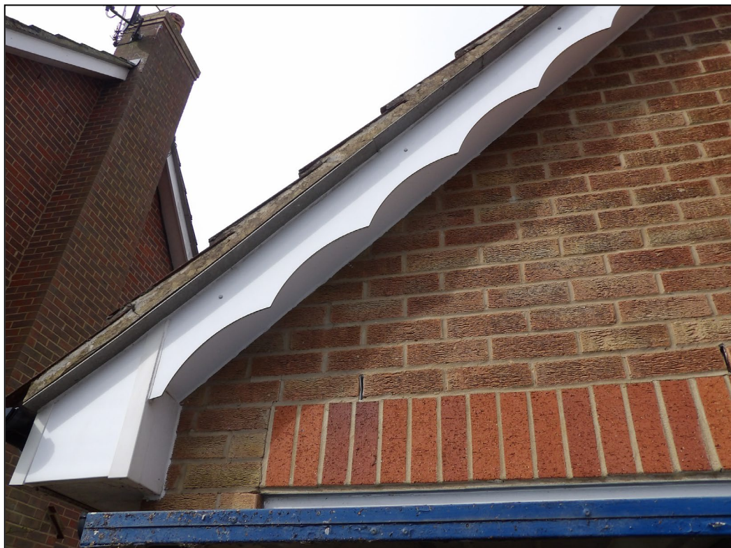
Figure 6. Example sealed uPVC soffits/fascias. 196 Hurricane Way, Woodley. 17.03.26
