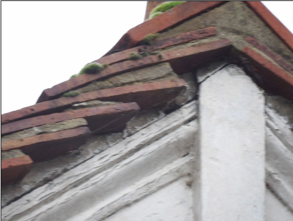
Figure 6. Well cemented verge on main property. Arlington, Basingstoke Road, Spencers Wood. 10.12.24
