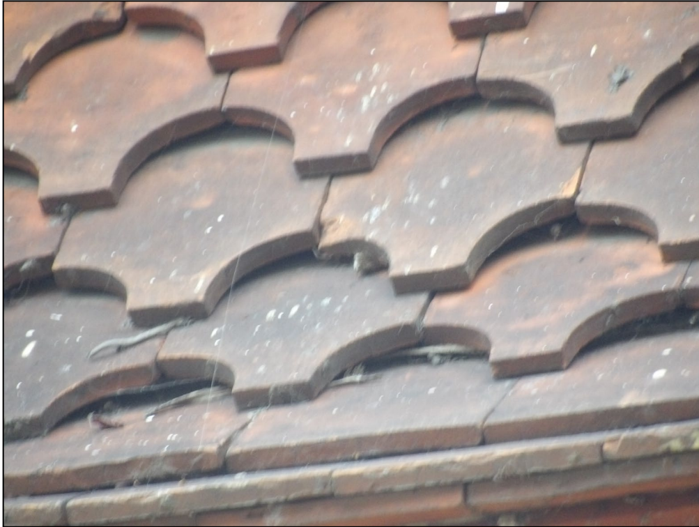
Figure 9. Example of gaps in hanging tiles. Arlington, Basingstoke Road, Spencers Wood. 10.12.24
