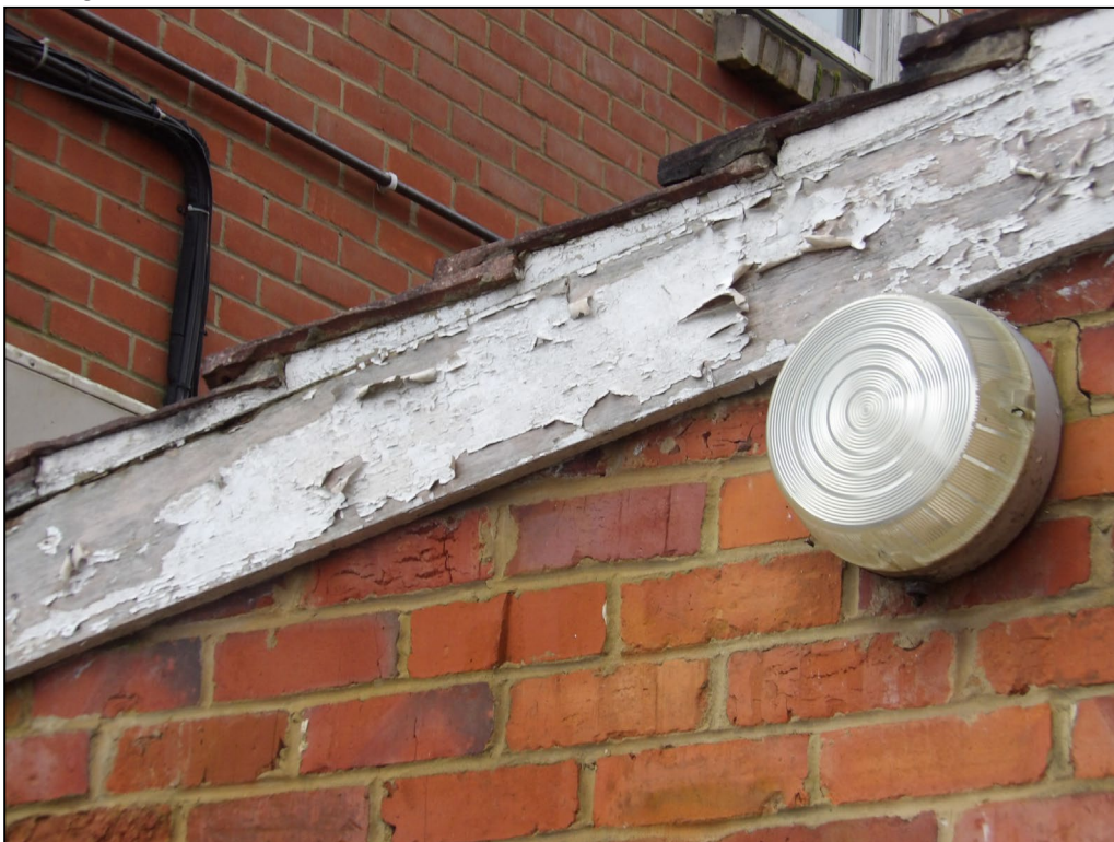
Figure 14. Example flush fascias and sealed verges on garage/utility. Arlington, Basingstoke Road, Spencers Wood. 10.12.24
