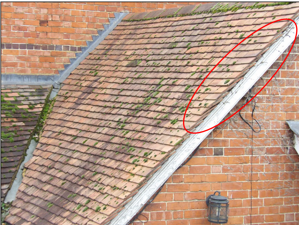
Figure 12. Gaps in verge of rear extension. Arlington, Basingstoke Road, Spencers Wood. 10.12.24
