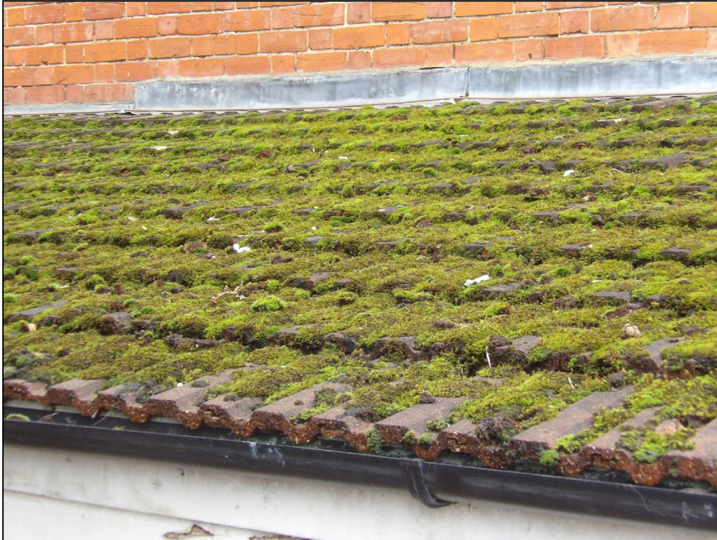
Figure 13. Example roof tiles on garage/utility and sealed flashing. Arlington, Basingstoke Road, Spencers Wood. 10.12.24
