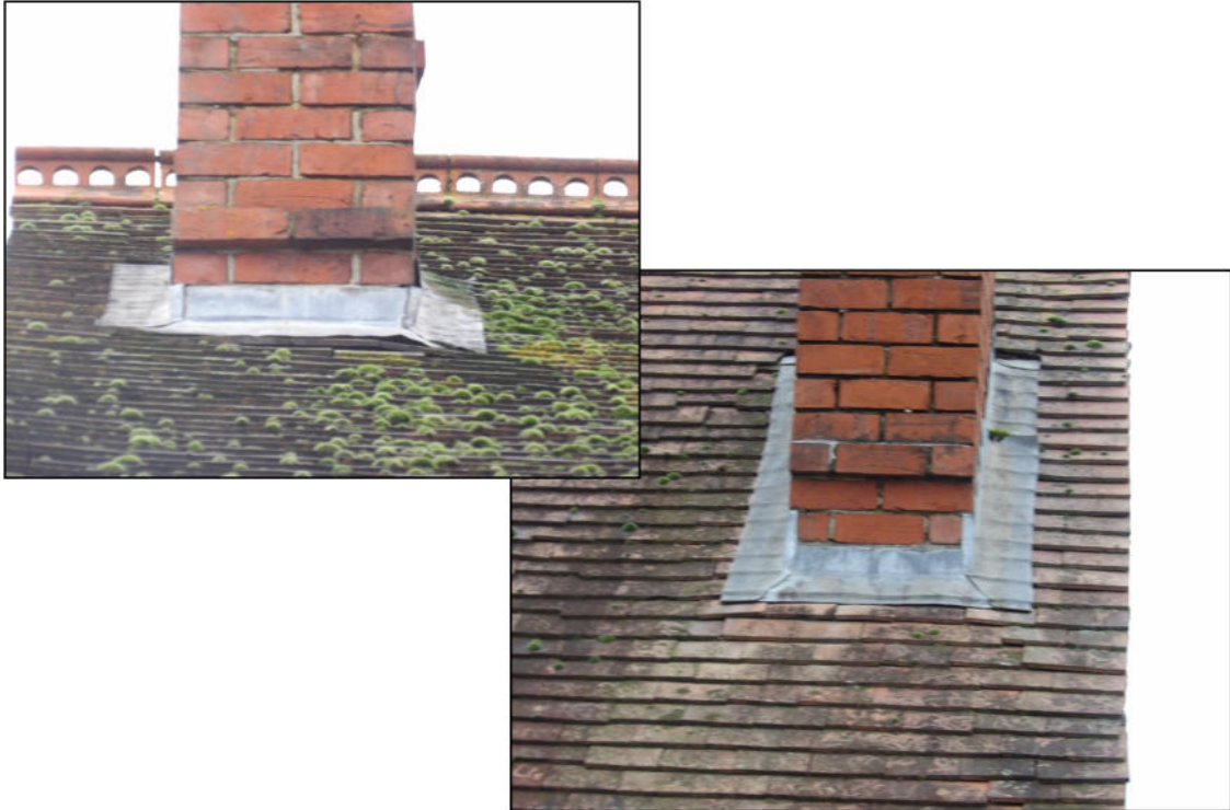
Figure 7. Example gaps in tiles/lead flashing around chimney stacks. Arlington, Basingstoke Road, Spencers Wood. 10.12.24
