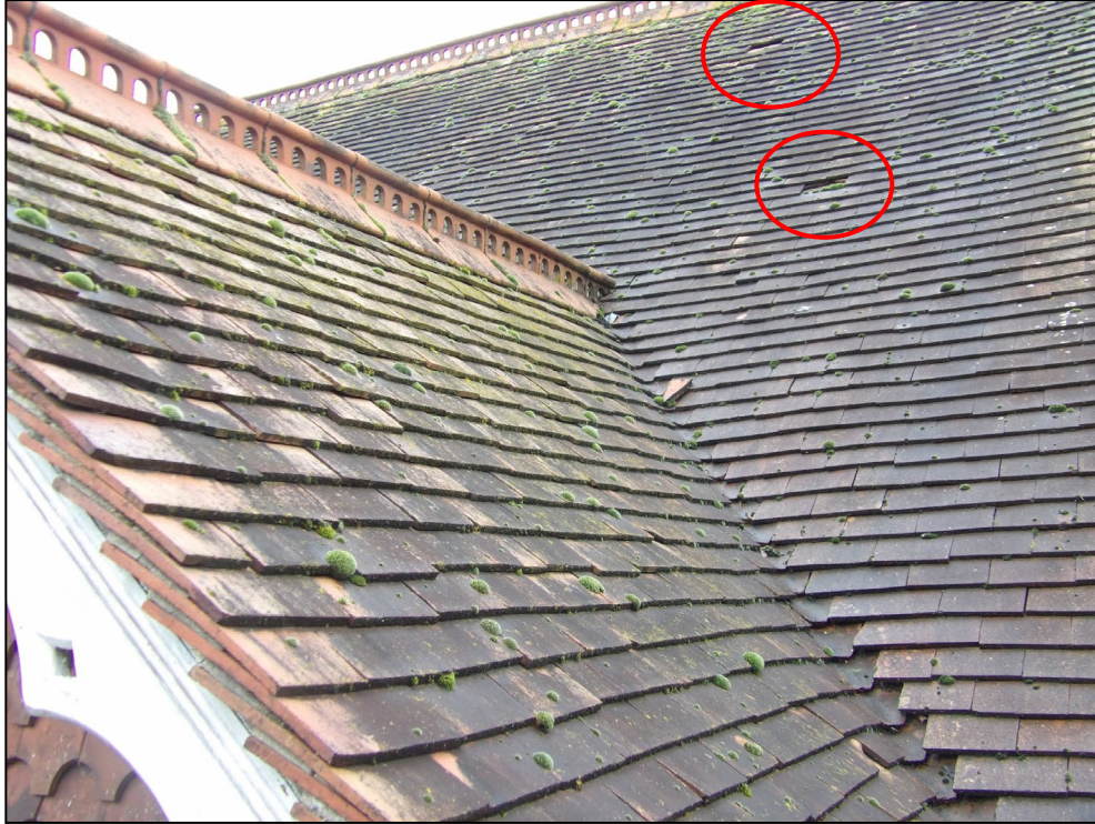
Figure 5. Missing roof/broken tiles. Arlington, Basingstoke Road, Spencers Wood. 10.12.24
