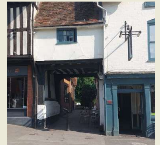
Figure 71: Typical covered passageway leading to courtyard
