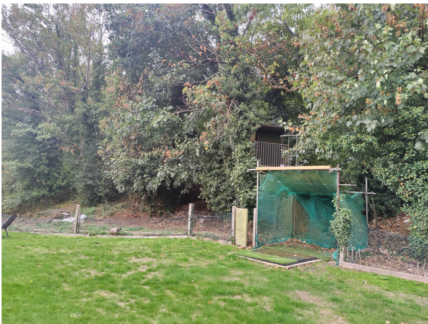
PHOTO 2: REAR BOUNDARIES (A) AND (B1)- UNAFFECTED BY EXTENSION WORKS CHICKEN WIRE MESH AND CONCRETE POSTS RESTORED TO GOOD ORDER
