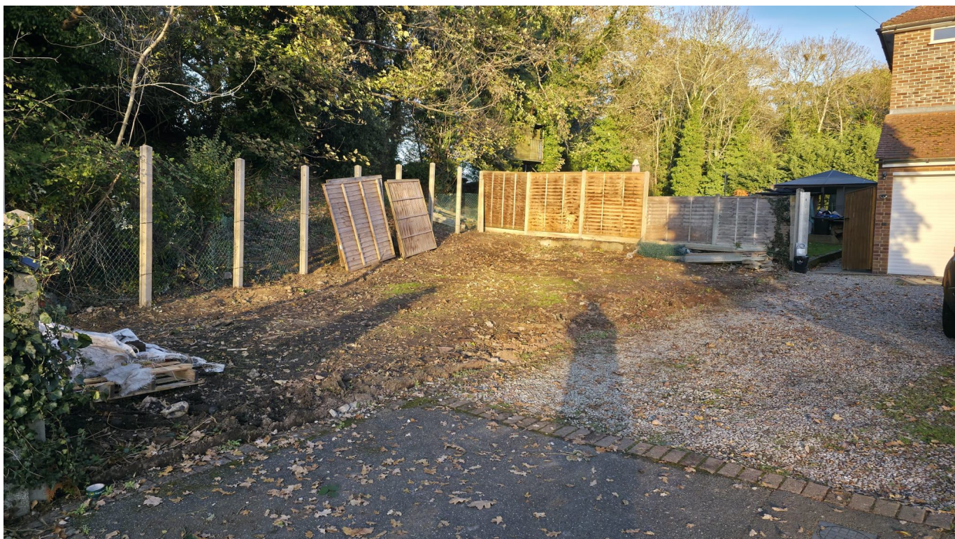
PHOTO 1: FRONT BOUNDARY (B2) – UNAFFECTED BY EXTENSION CHICKEN WIRE MESH AND CONCRETE POSTS RESTORED TO GOOD ORDER
