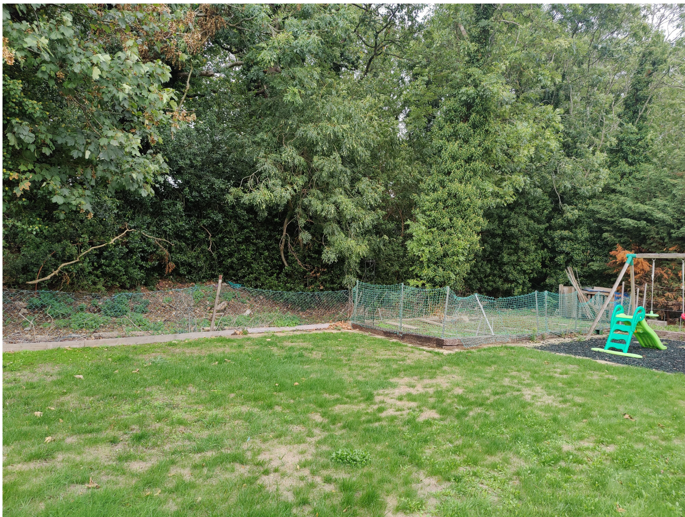
PHOTO 3: REAR BOUNDARIES (A) AND (B1)- UNAFFECTED BY EXTENSION WORKS CHICKEN WIRE MESH AND CONCRETE POSTS RESTORED TO GOOD ORDER
