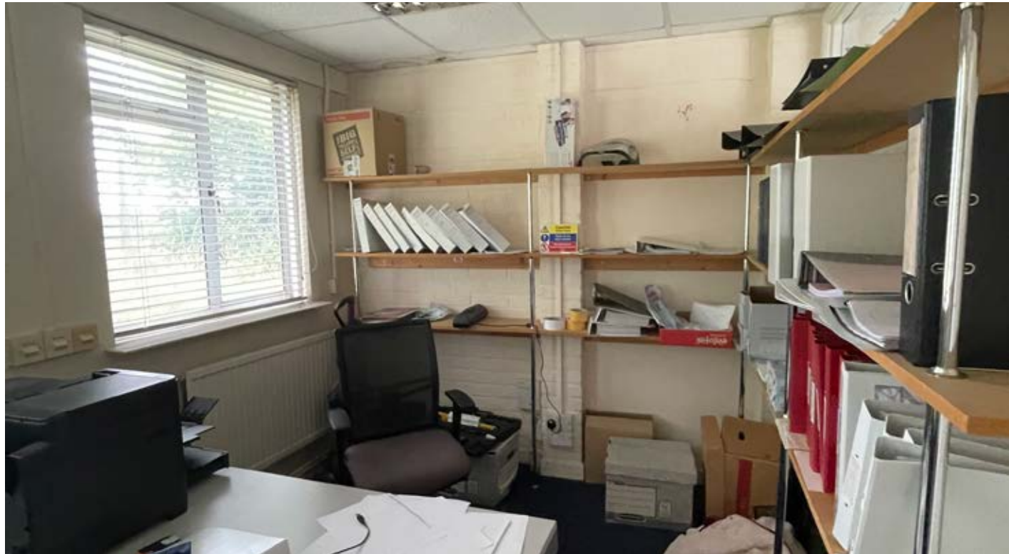
Internal form of east wing with modern inserted ceiling shown
