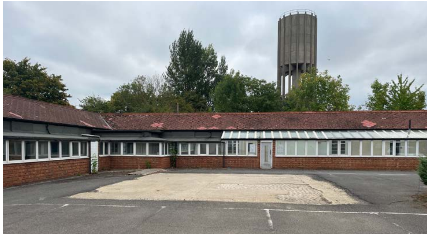
East External Wing with modern PVC extension shown
