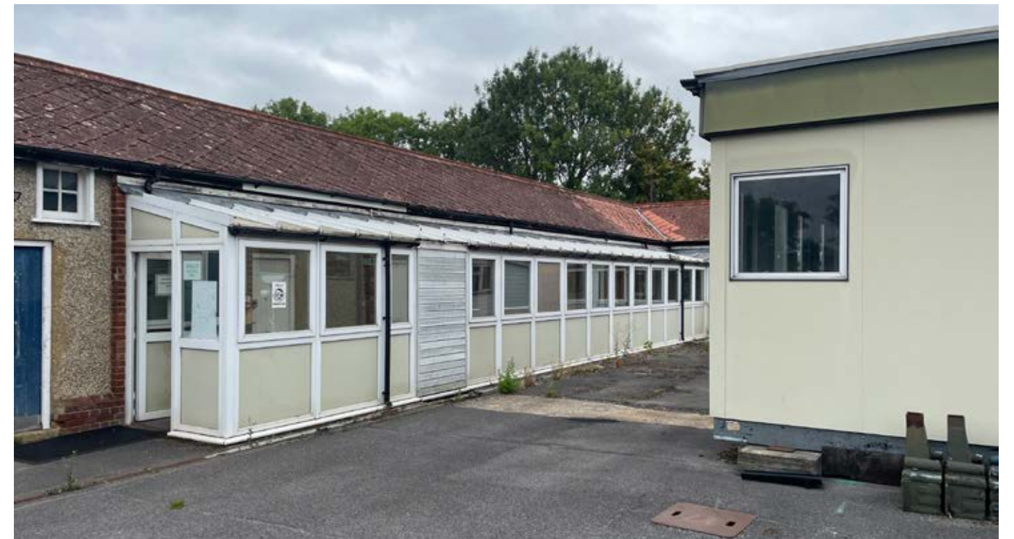
East External Wing with modern PVC extension shown
