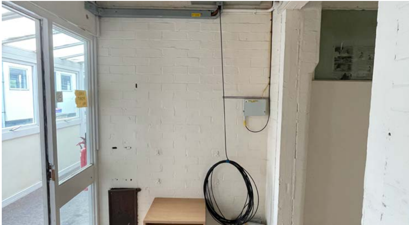
Internal form of west wing with modern partitions and primary brick wall shown
