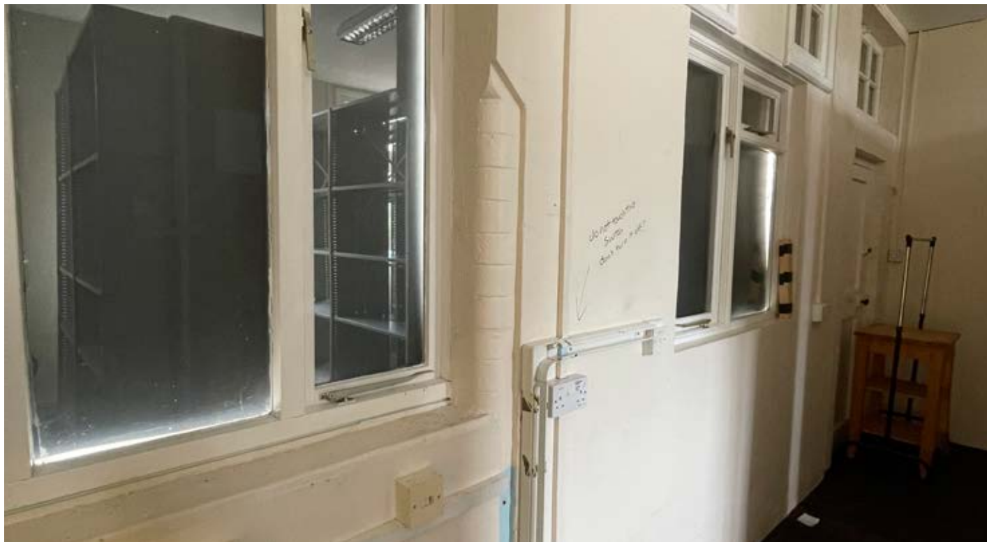
Internal form of west wing showing primary external wall with inserted windows
