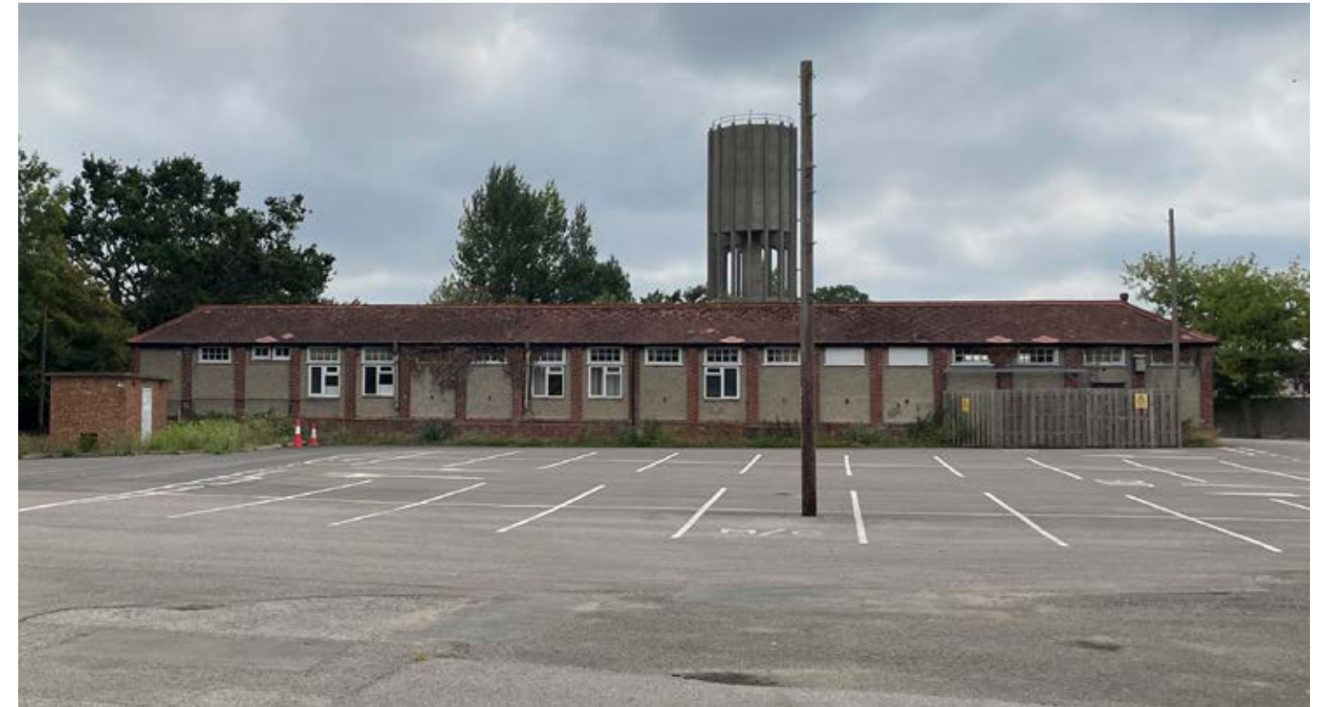
West External Elevation with numerous modern PVC window openings shown
