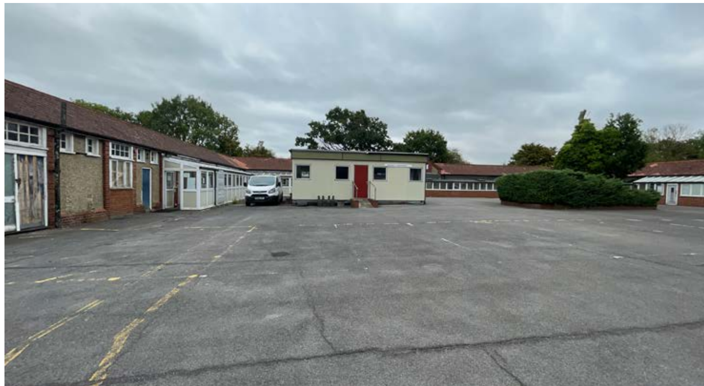
East and North External Wing with modern PVC extension and central modern out building shown
