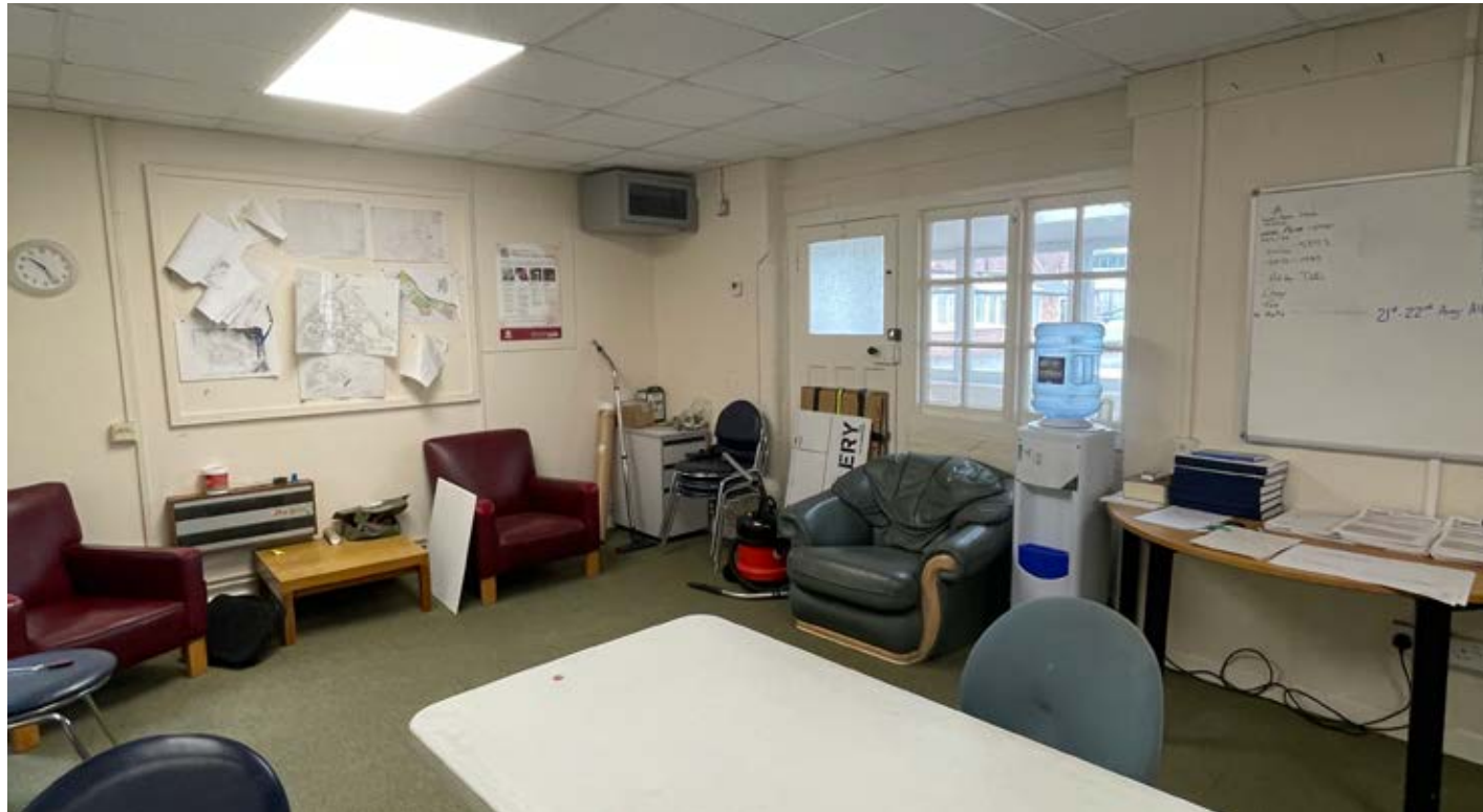
Internal form of north wing with modern inserted ceiling shown
