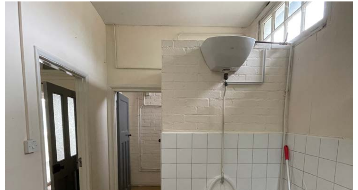
Internal form of west wing showing remains of a primary partition in the context of the modern use of the space and secondary partitions
