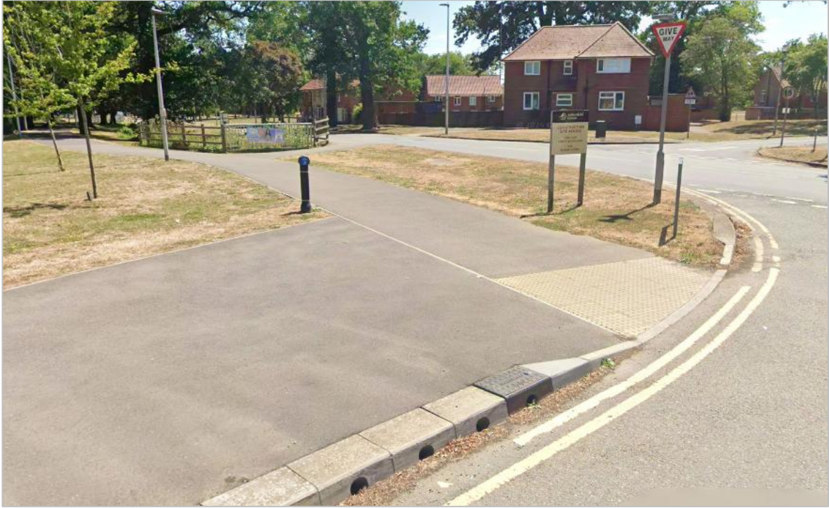
Image 2.2: Shared footway / cycleway provision along Biggs Lane
