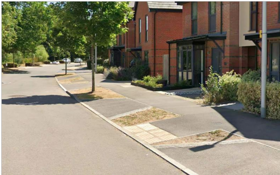
Image 2.12: Footway provision along Princess Marina Drive
