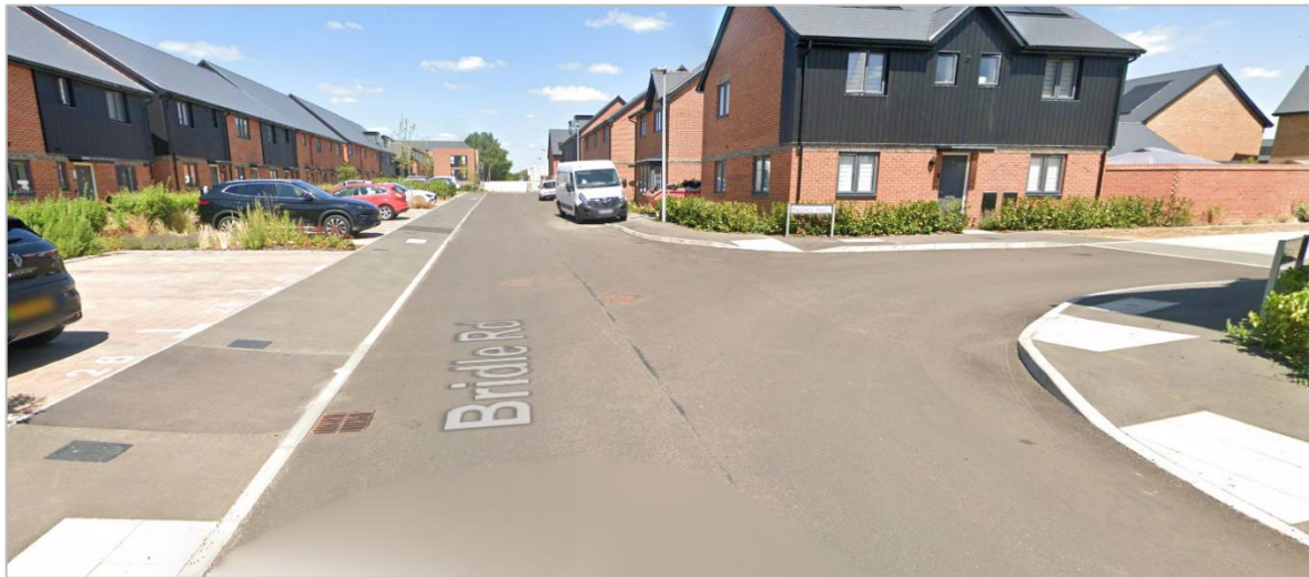
Image 2.3: Footways on Bridle Road
