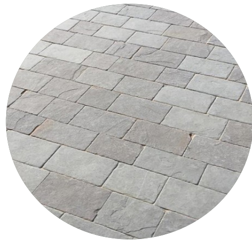
Shared Surfaces Block Paving
