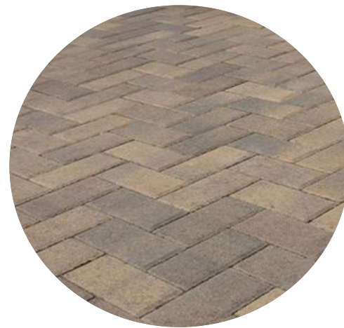
Parking Surface Permeable Block Paving
