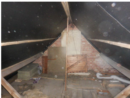
Photograph 9. Roof void showing boarded floor and felt fixed to the underside of the rafters.
