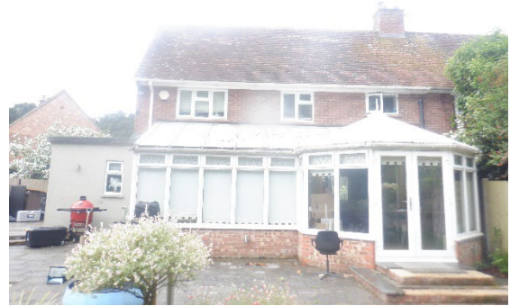
Photograph 2. Rear of property viewed from south.
