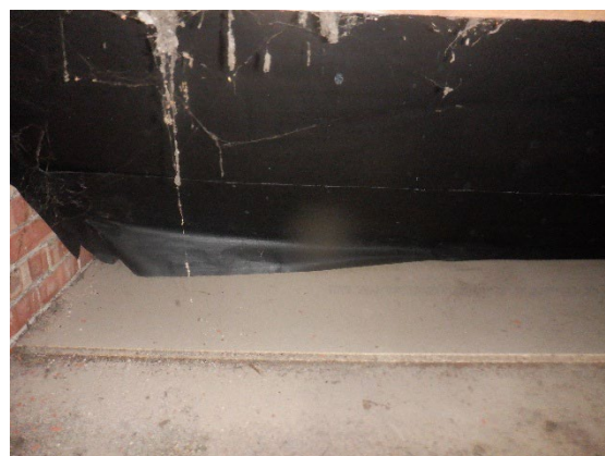
Photograph 12. Felt extending down to the eaves.
