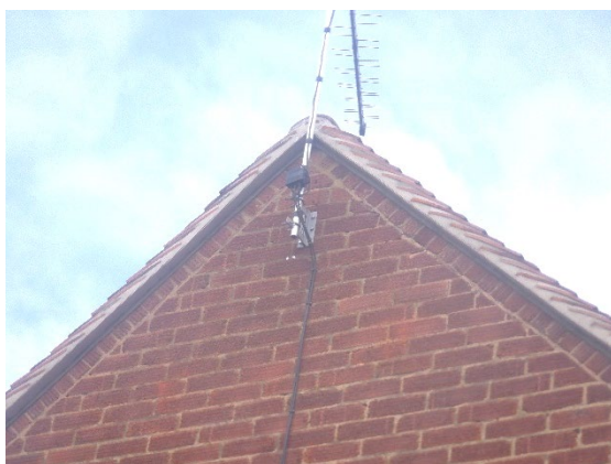
Photograph 5. Recently re-bedded verge mortar (side (north western) elevation).
