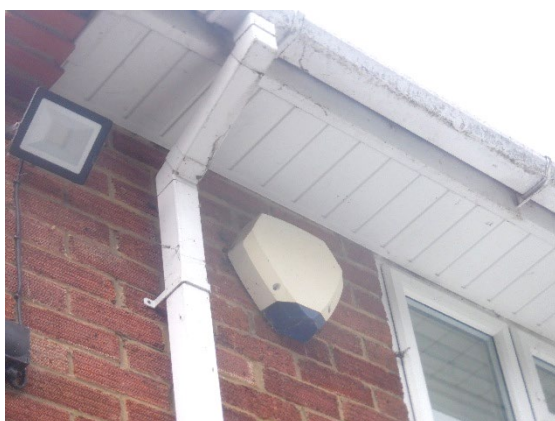
Photograph 7. Tightly fitted uPVC soffits (rear elevation).
