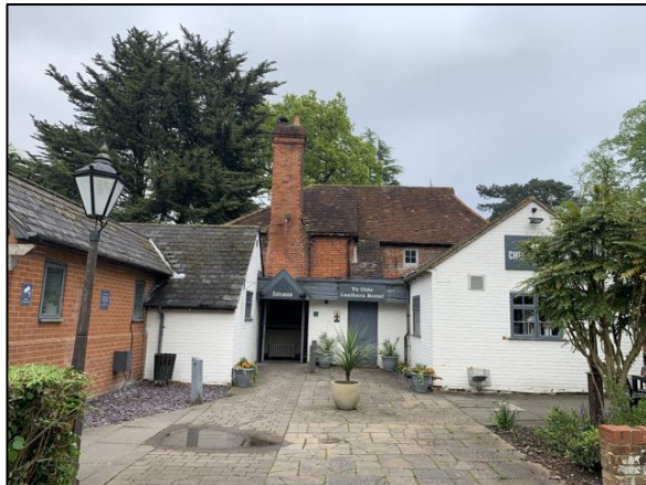
Photo 35 W elevation, older section
