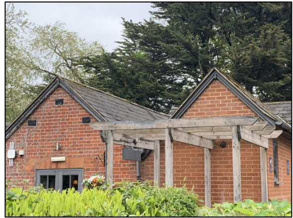
Photo 36 W elevation, newer section
