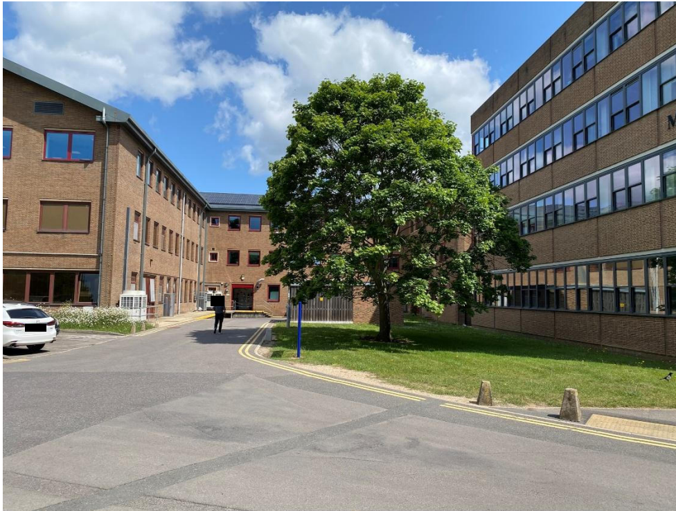
Photo 1 – Loading bay to rear of JJ Thomson Building and substation as seen from road 2 nd Avenue.
