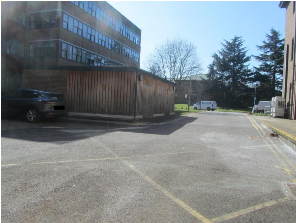
Photo 3 – Substation as seen from loading bay to rear of J J Thomson Building
