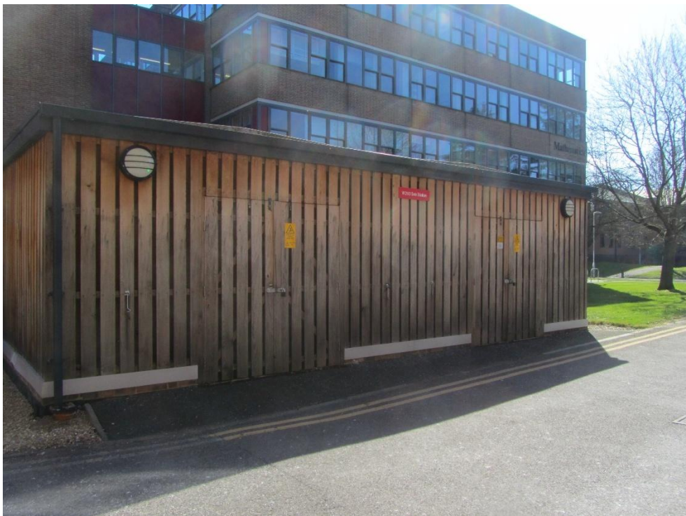
Photo 4 – Front elevation of existing substation
